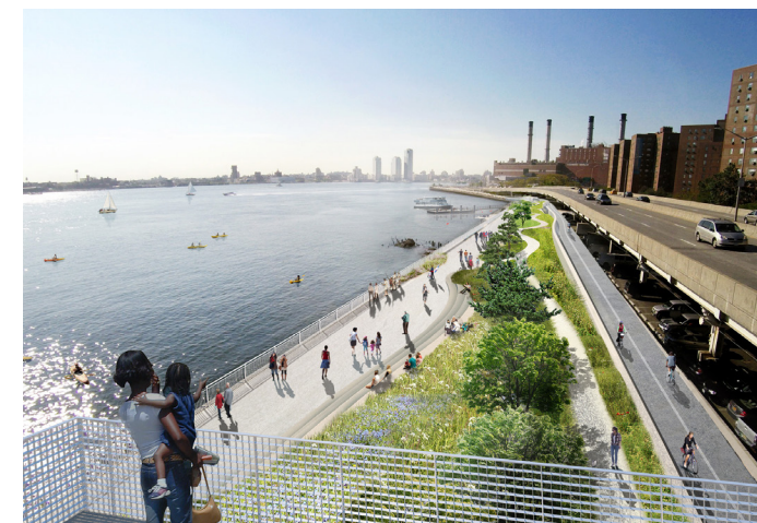
Rendering of East Side Coastal Resiliency project, a resilient park along East River that will be elevated to protect against 2050s storm surge.
