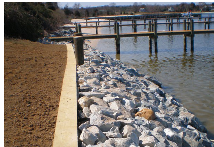
Example of a low raised edge using revetment.
