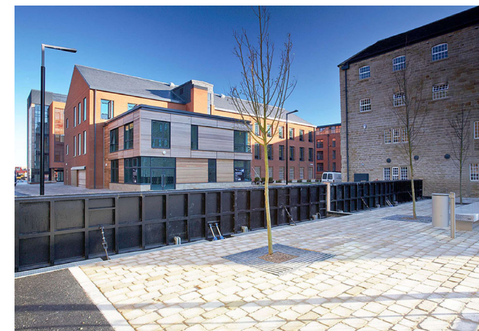
Example of small-scale deployable protection in the form of flip-up barriers. In normal conditions, flip-up barriers would be flipped down and hidden.
