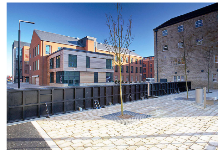
Example of small-scale deployable protection in the form of flip-up barriers. In normal conditions, flip-up barriers would be flipped down and hidden.
