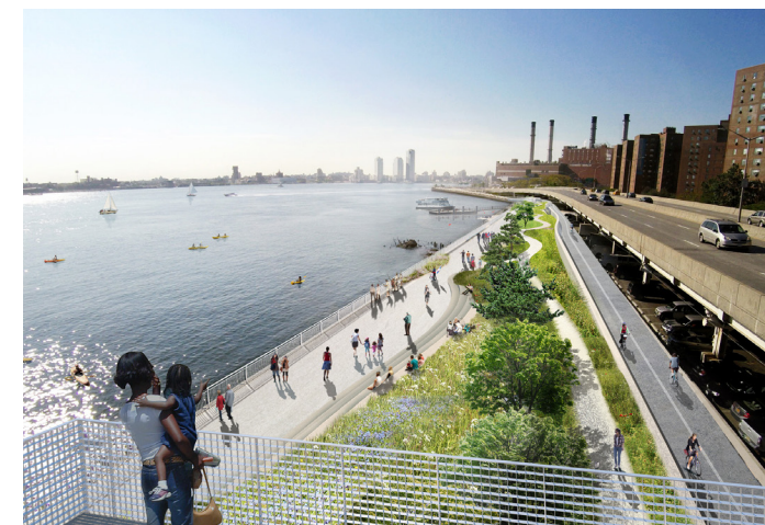
Rendering of East Side Coastal Resiliency project, a resilient park along East River that will be elevated to protect against 2050s storm surge.
