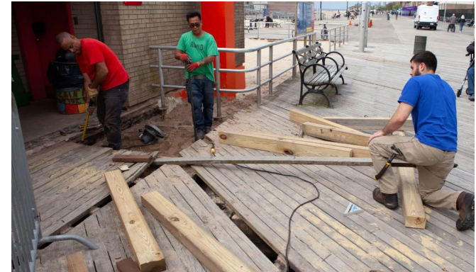
NYC Parks carpenters repair deck planks
