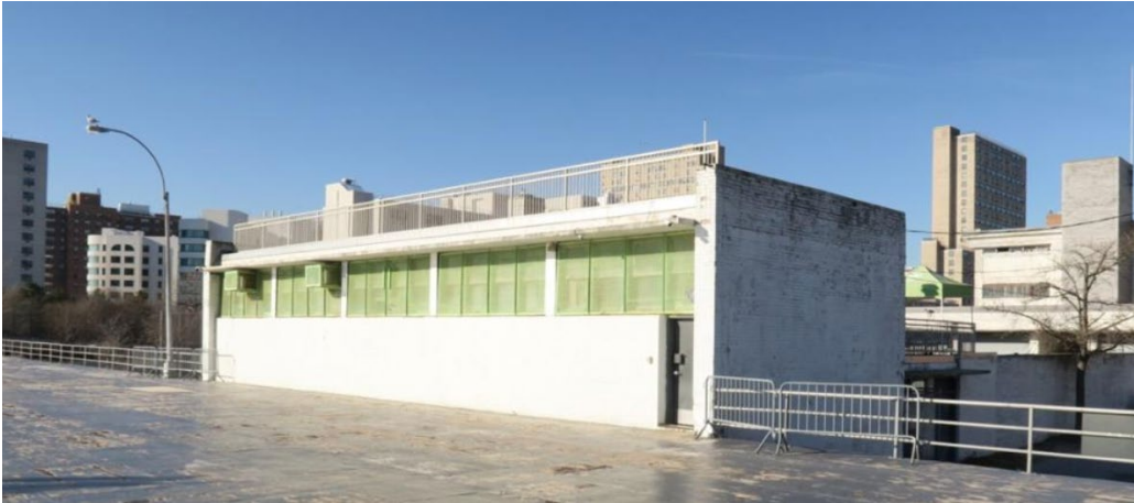
Parks garage building
