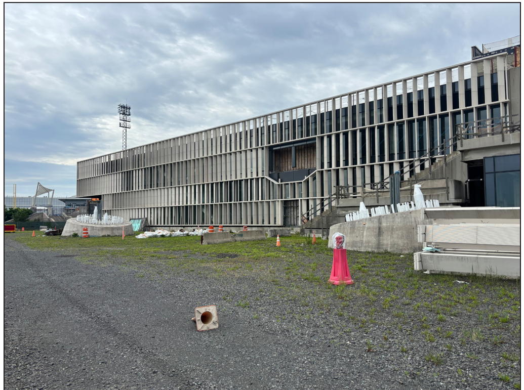
View looking south from within Site 2 towards the terminal building
