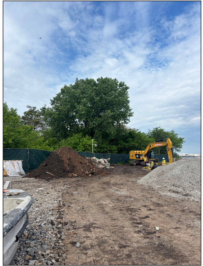
View looking west towards Site 3 13
