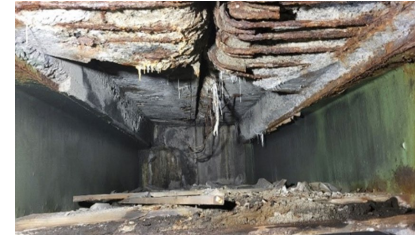
Columbia Heights Bridge underdeck
