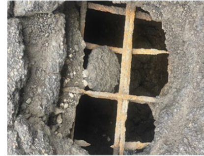
Deck through holes over Old Fulton Street
