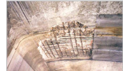
Typical joint condition along the triple cantilever
