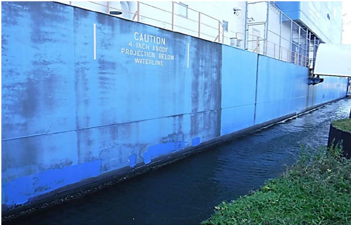
Photo 4.1-1: Typical condition of the hull coating along the waterline.
