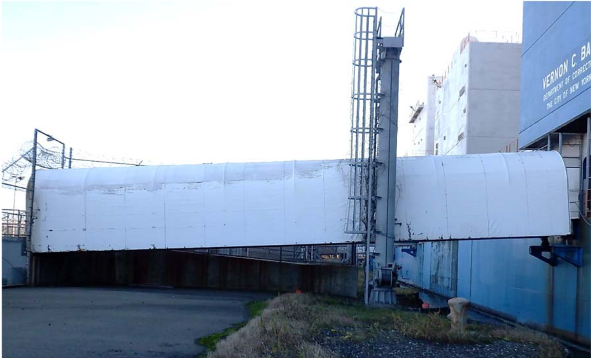
Photo 3.7-5: West elevation view of the Middle Gangway B and support frame. Note the vines growing on the support frame stairs.
