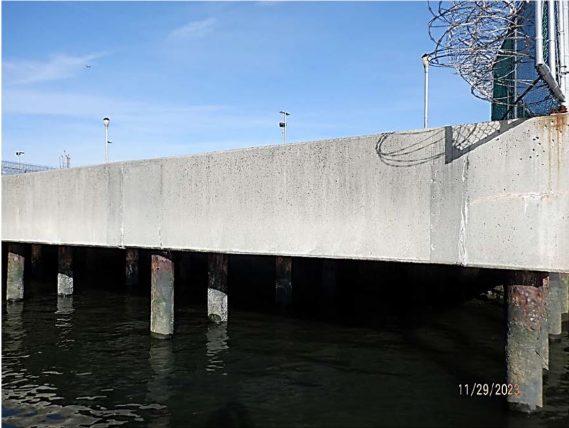
Photo 3.3-4: Elevation view of the edge beam along the High-Level Platform.
