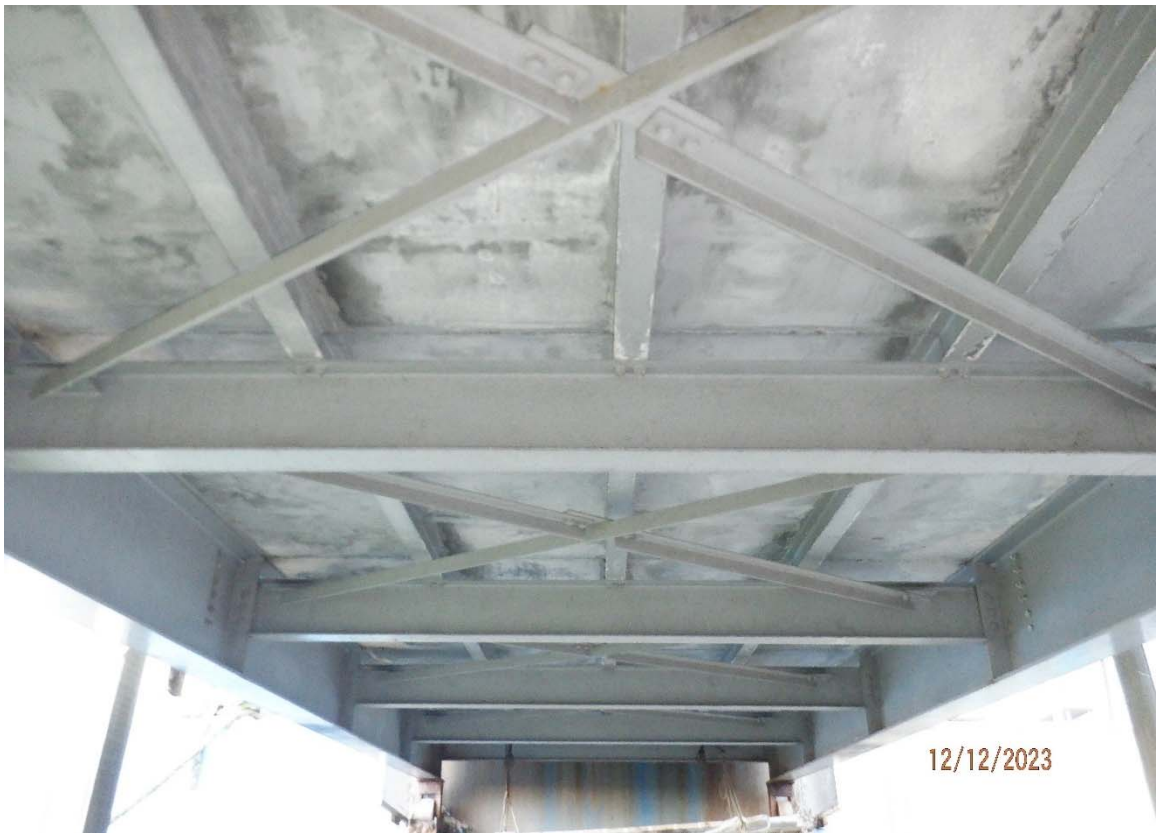
Photo 3.9-2: View of the Cargo Gangway framing looking south.
