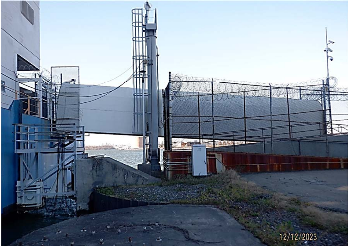
Photo 3.6-1: Overall east elevation view of the West Pedestrian Gangway A and the gangway support frame.
