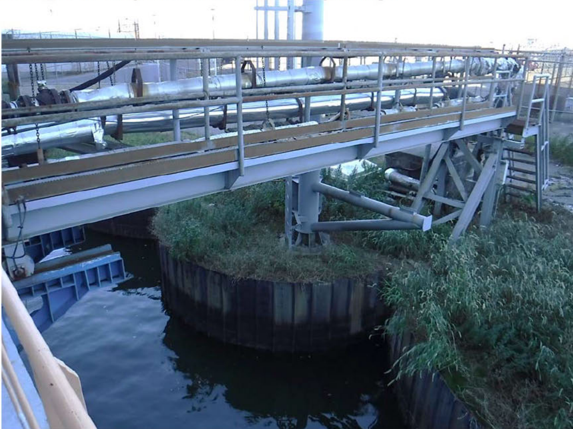
Photo 3.10-5: View of the catwalk railing and steps looking north.
