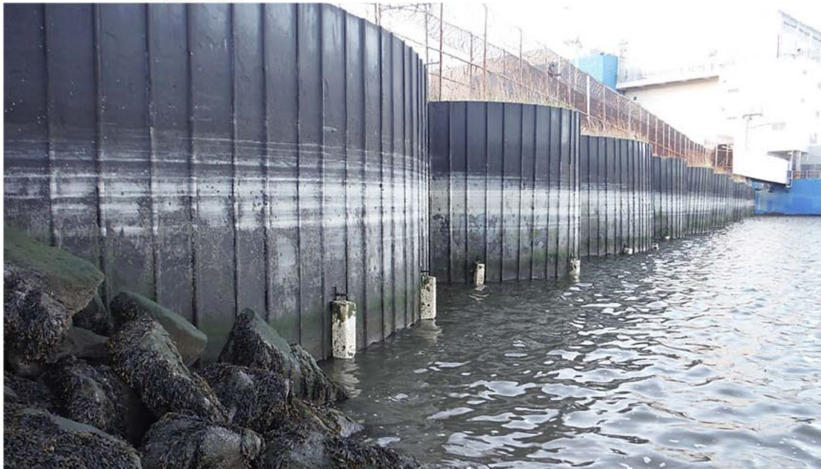
Photo 3.1-1: Overall view of the cellular steel sheet pile cofferdam (west leg) as viewed from Cell 25 looking south. Note the anodes above the water's surface.
