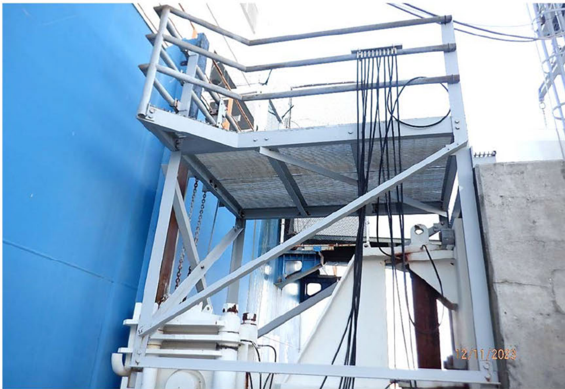
Photo 3.4-6: Overall view of the catwalk at the West Mooring Arm.
