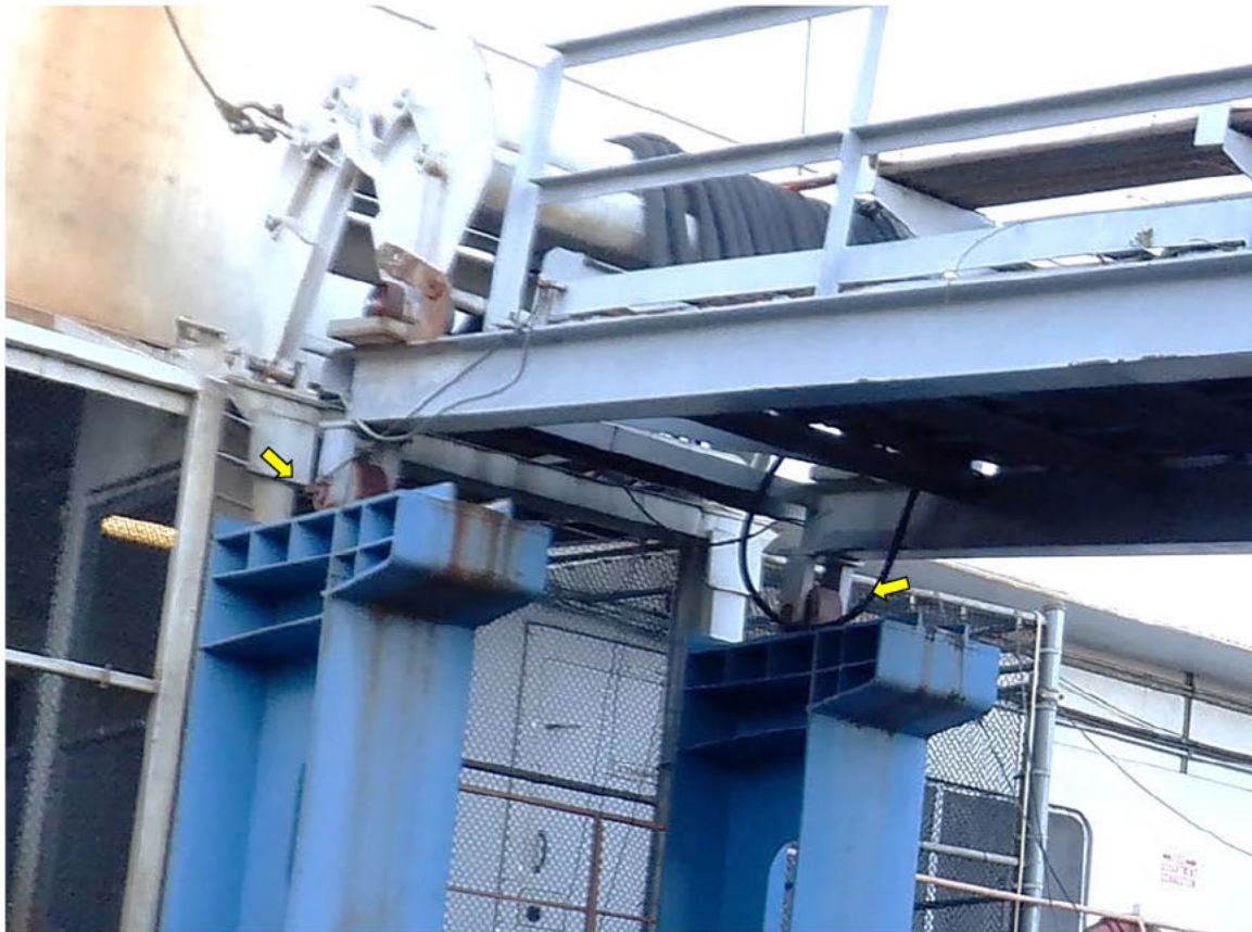
Photo 3.11-2: Enlarged view of the roller wheel bearings at the Electrical Gangway.
