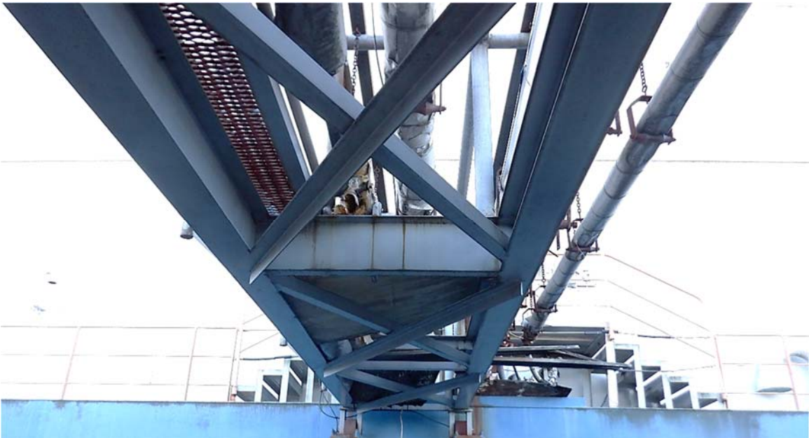
Photo 3.10-2: View of the Plumbing Gangway framing.
