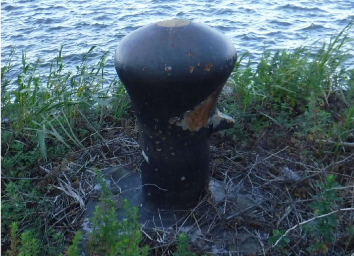
Photo 3.1-6: Bollard B-1 is inaccessible due to the security fence. Note the typical minor coating loss and surface rust.
