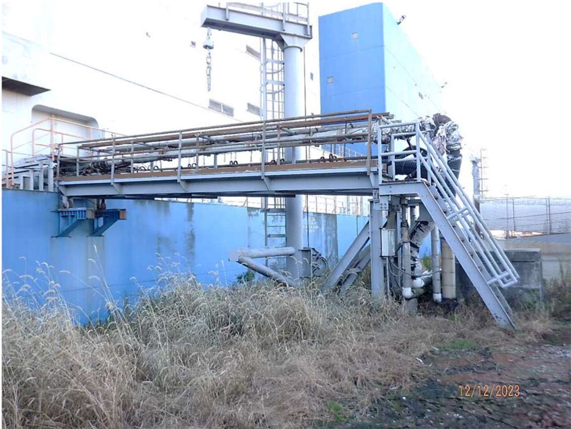
Photo 3.10-1: Overall view of the Plumbing Gangway.
