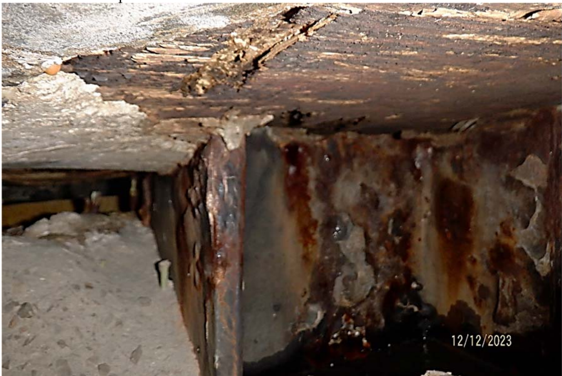
Photo 3.5-7: View of the northwest steel batter H-pile between the bottom of the pile cap and the top of the encasement.
