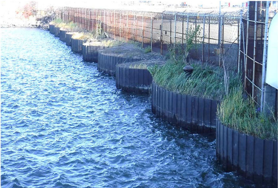
Photo 3.1-2: Overall view of the cellular steel sheet pile cofferdam (west leg) as viewed from Cell 15 looking north.
