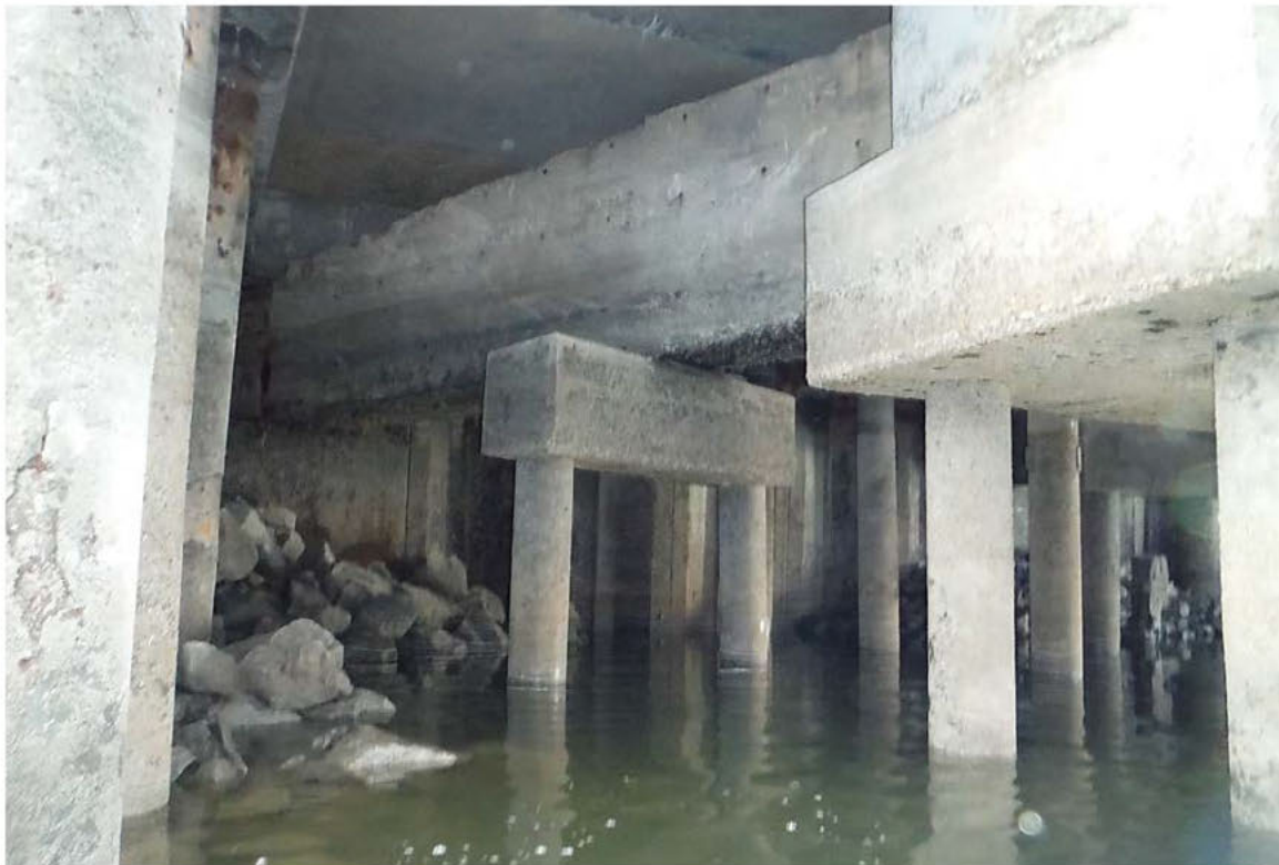
Photo 3.5-9: Typical condition of diagonal strut that braces the double-leg mooring arm pile cap.
