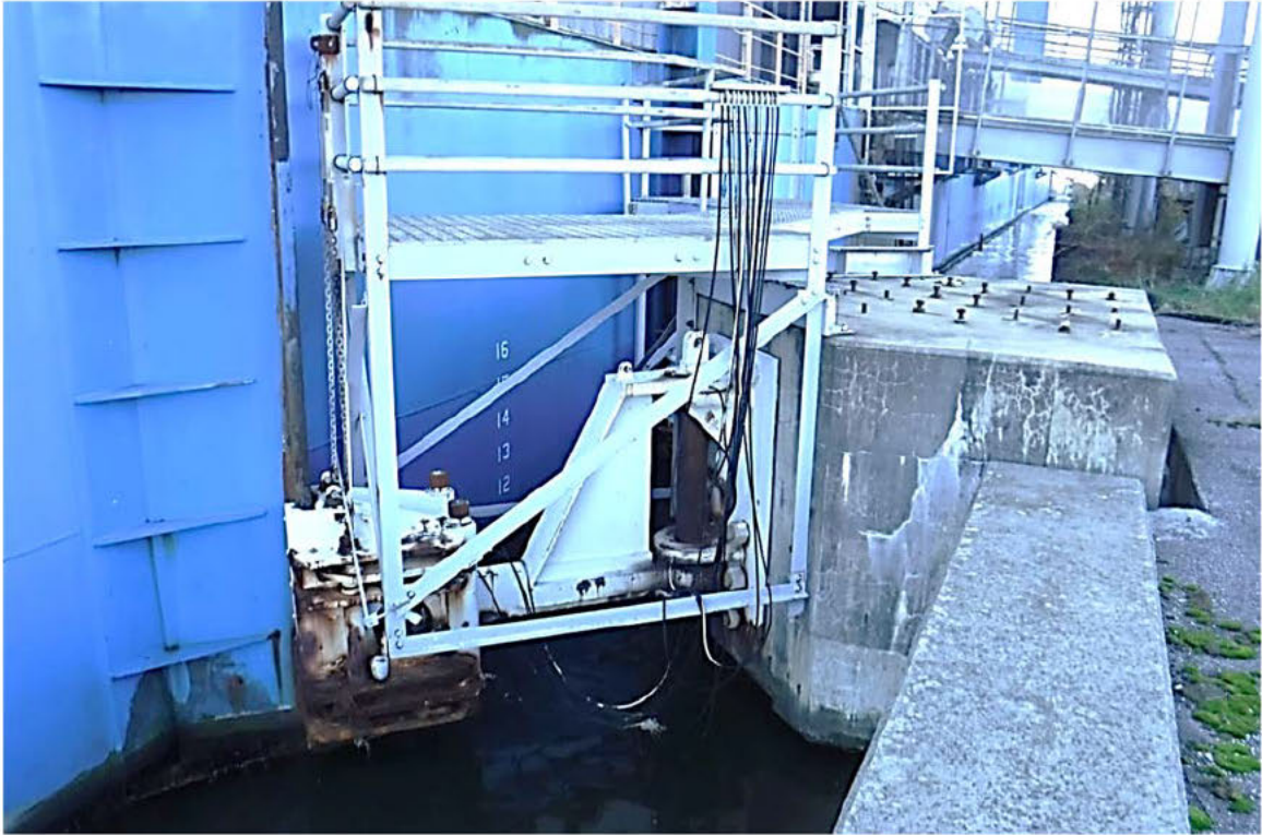
Photo 3.5-1: Overall view of the east leg of the East Mooring Arm.
