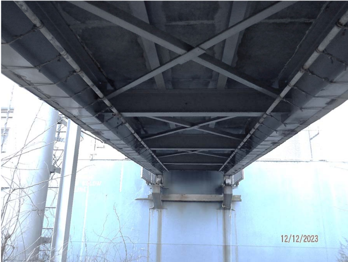
Photo 3.8-1: View of the framing underside and roller bearing supports at the East Pedestrian Gangway C.
