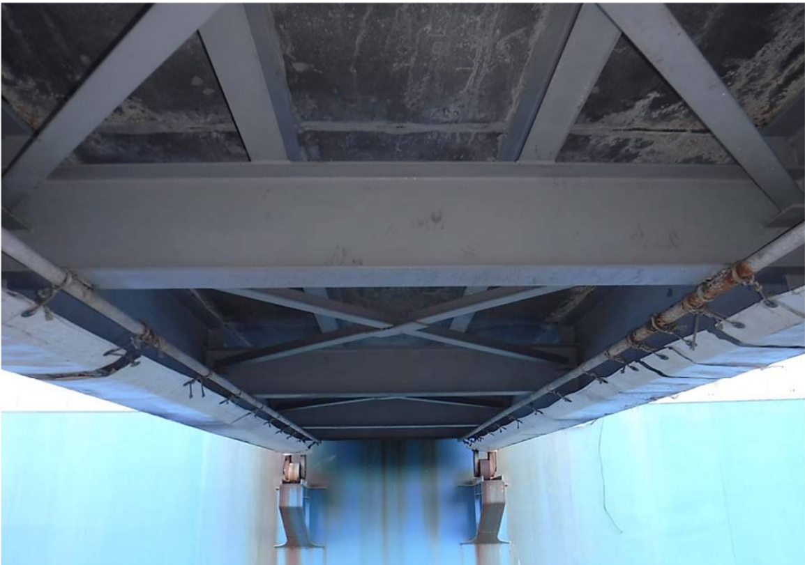
Photo 3.7-2: View of the Middle Pedestrian Gangway B framing looking south.
