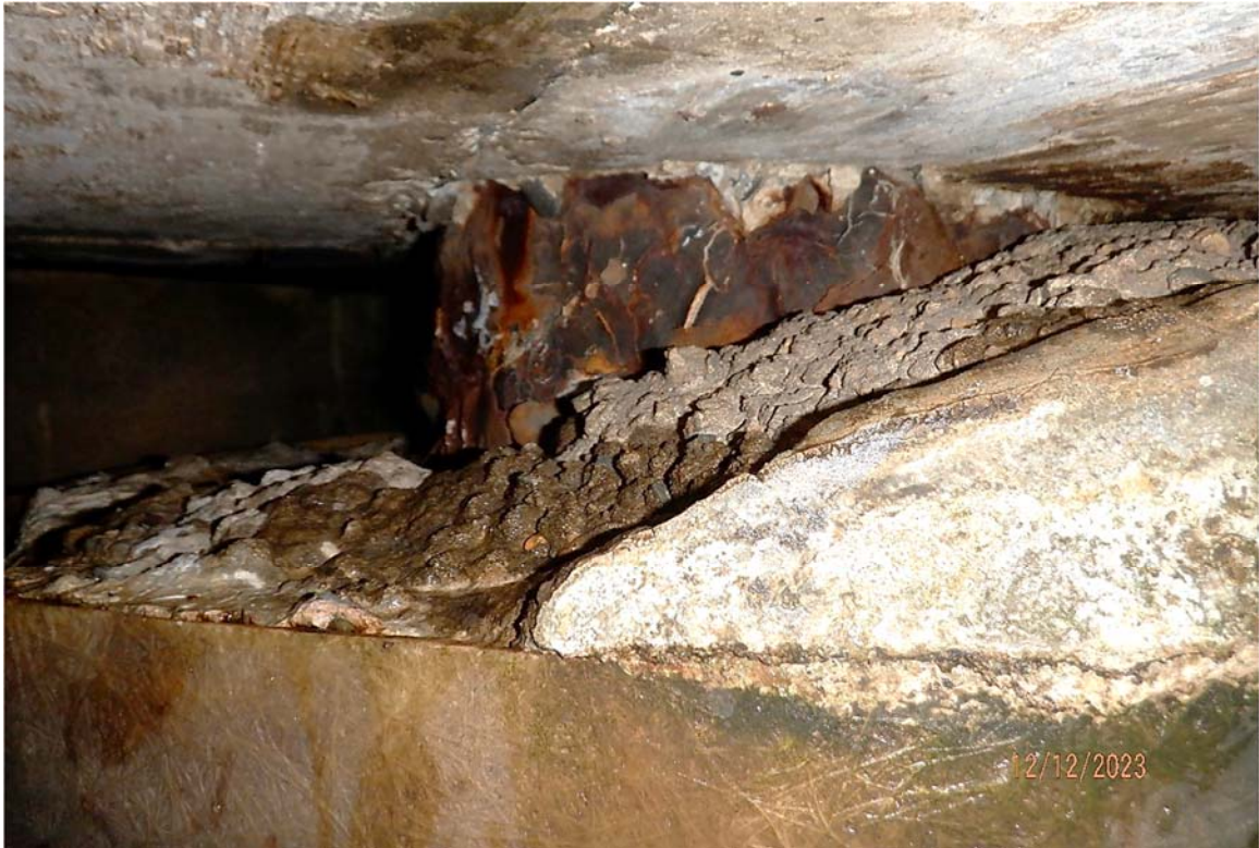
Photo 3.5-6: View of the southeast steel pipe pile between the bottom of the pile cap and the top of the encasement.
