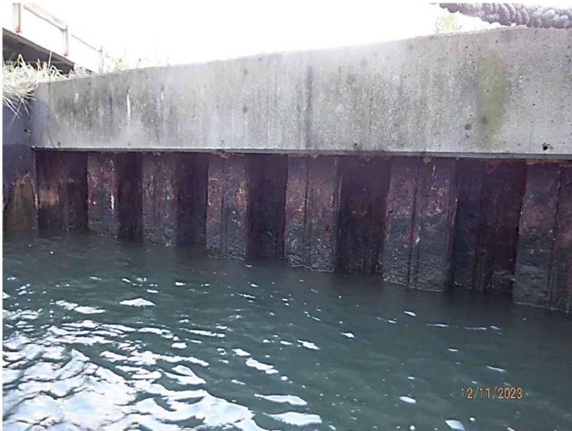
Photo 3.2-3: Elevation view of the concrete pile cap at the Transition Bulkhead.
