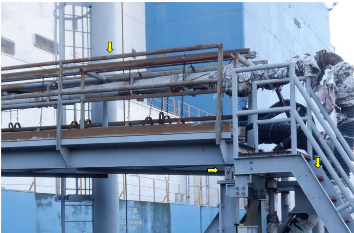
Photo 3.10-4: Enlarged view of the catwalk railing and steps.
