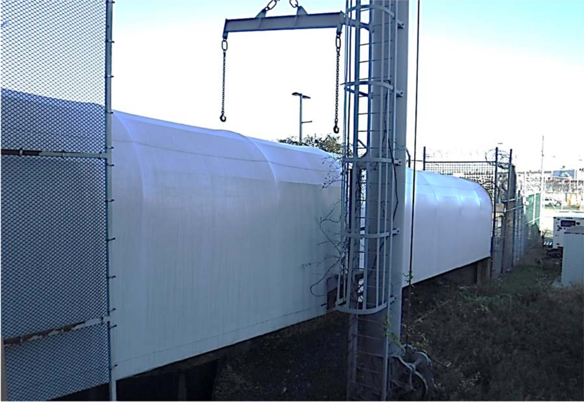
Photo 3.8-4: Overall east elevation view of the East Pedestrian Gangway C and the gangway support frame.
