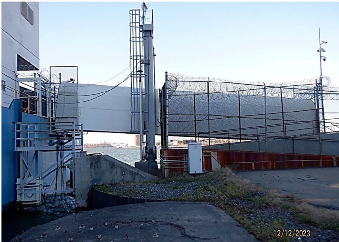
Photo 3.6-7: Overall east elevation view of the West Pedestrian Gangway A and the gangway support frame.
