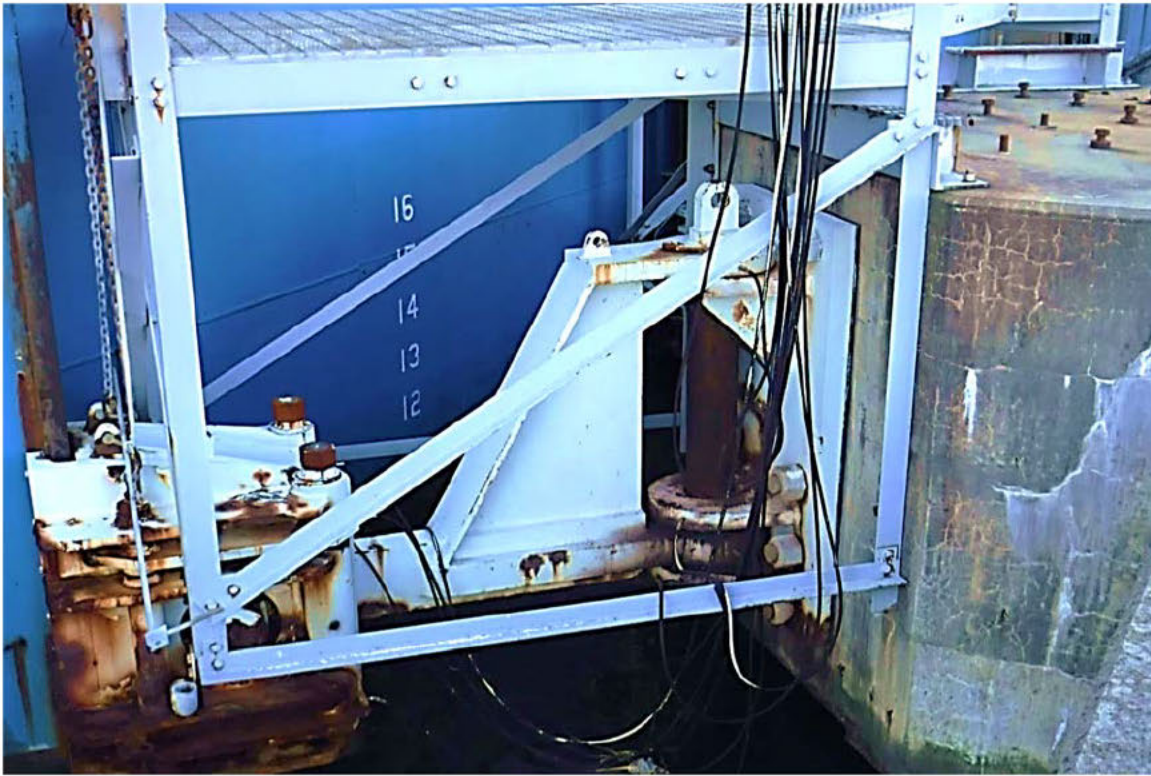
Photo 3.5-3: Overall view of the west leg of the East Mooring Arm.
