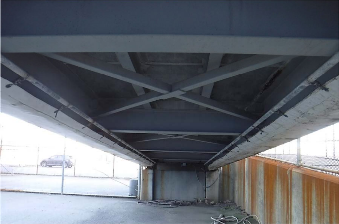
Photo 3.7-1: View of the Middle Pedestrian Gangway B framing looking north. The coating generally remains intact.
