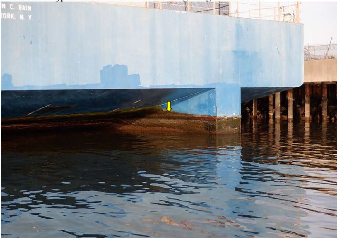
Photo 4.1-2: Loss of coating with minor corrosion along the waterline at the east rake of the barge.
