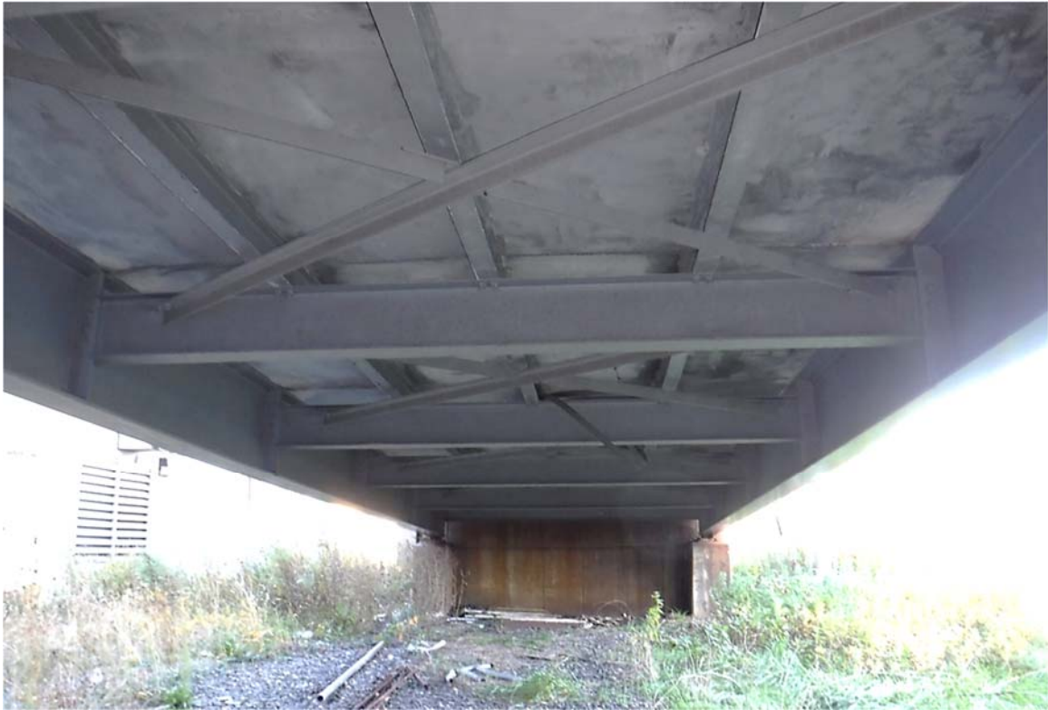
Photo 3.9-1: View of the Cargo Gangway framing looking north.
