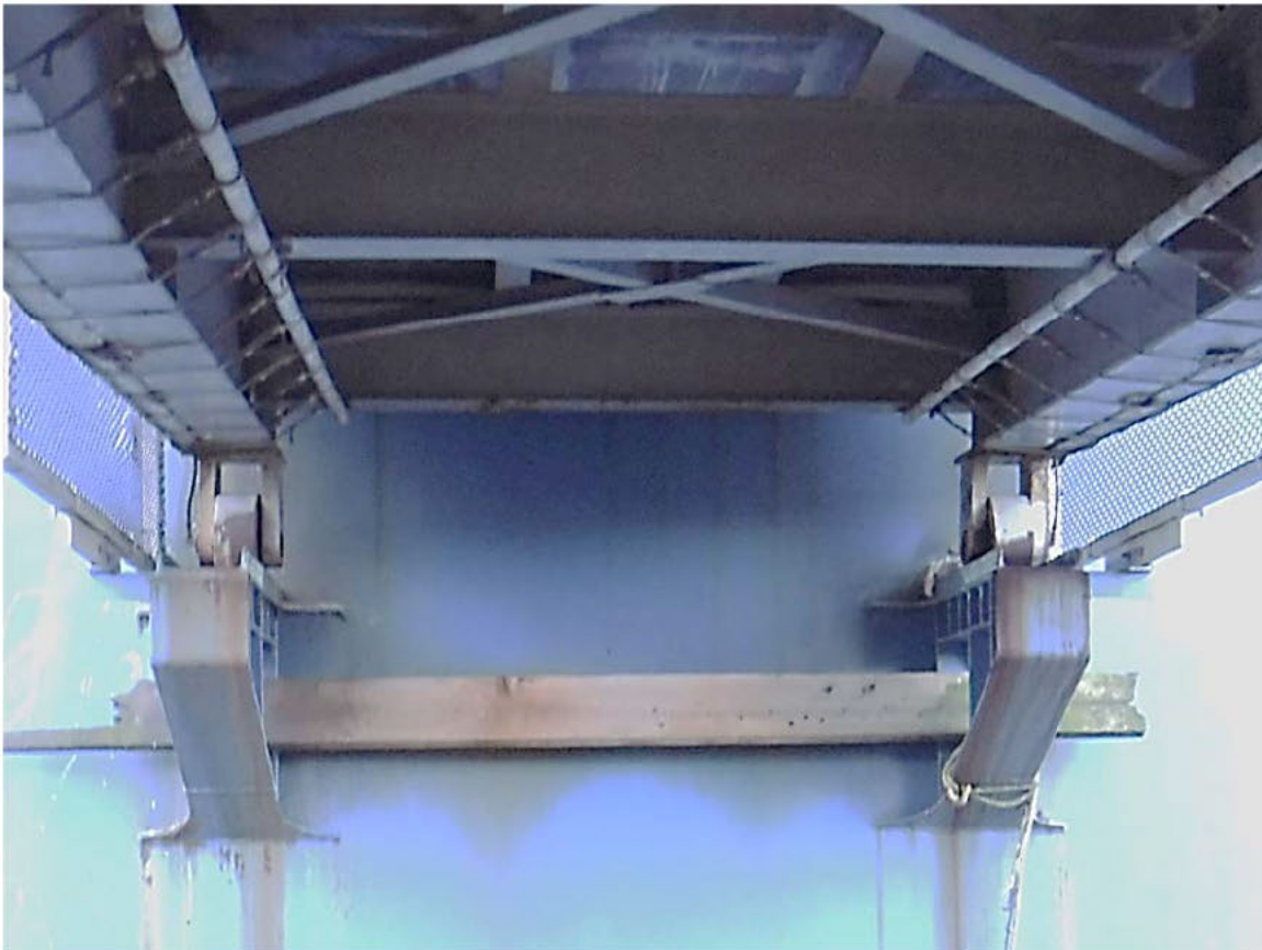
Photo 3.8-2: View of the roller bearings at East Pedestrian Gangway C.
