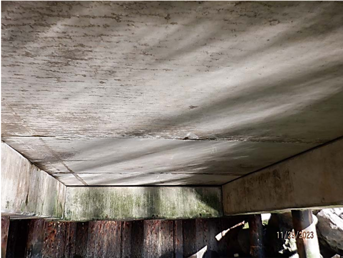
Photo 3.3-5: Typical condition of the precast concrete deck underside.
