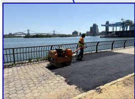
94 th street sinkhole repair
