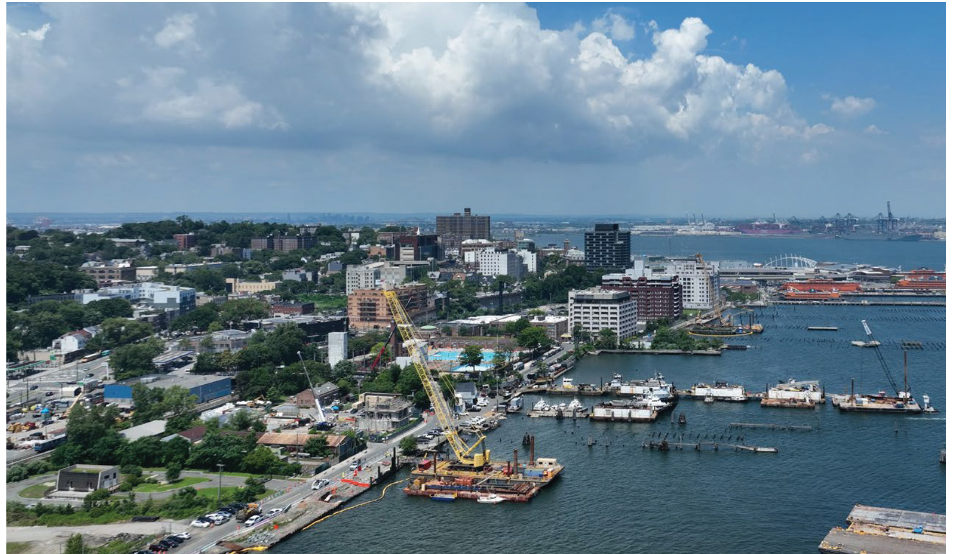
Construction along the Tompkinsville Esplanade.
