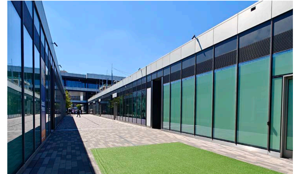
Empire Outlets: Empty Stores at Upper Level
