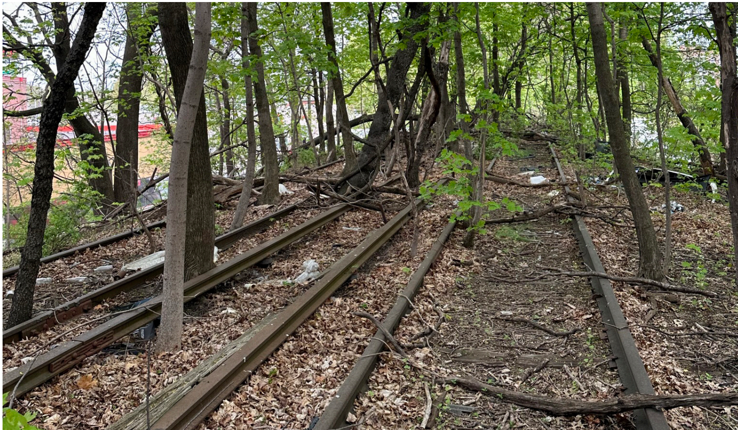
5 - Looking North from Top of the Embankment
