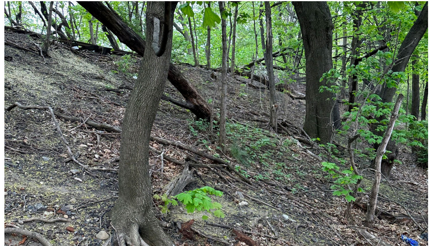
6 - Looking South East at Side Slope of the Embankment
