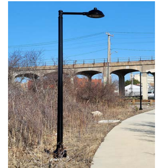
DOT-SL Standard Flushing Meadows Park Post with LED Stad Luminaire Mounted on Arm: Black
