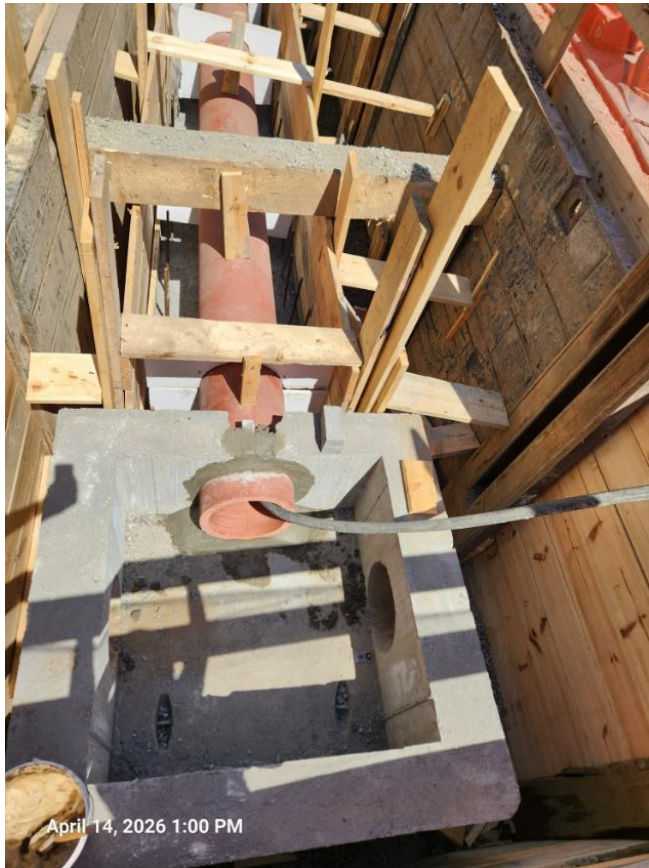
Storm Sewer Pipe Installation April 2026
