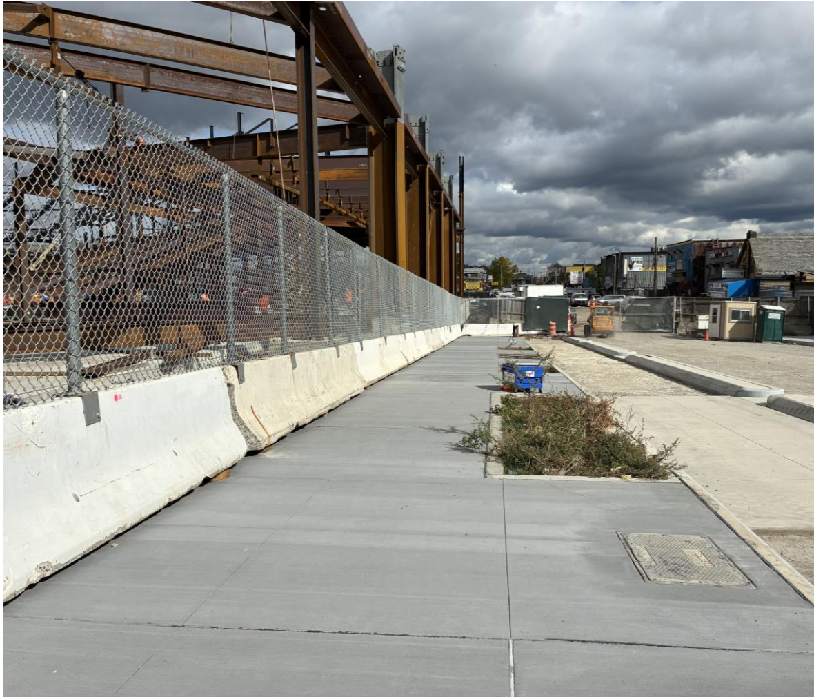
Willets Point Boulevard Sidewalks October 2025
