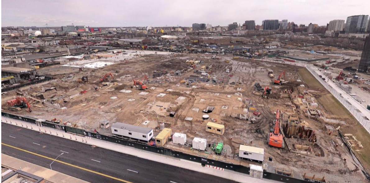
Aerial photo of stadium work site: April 2025
