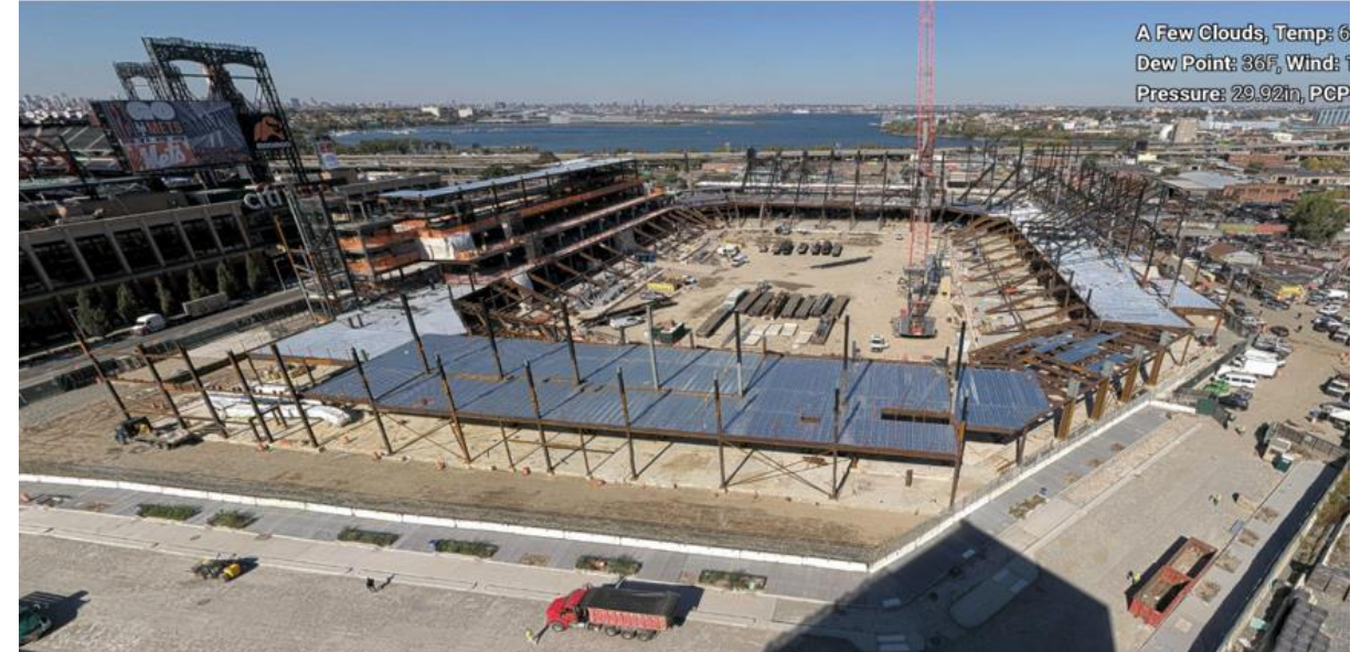
Aerial photo of stadium work site: October 2025
