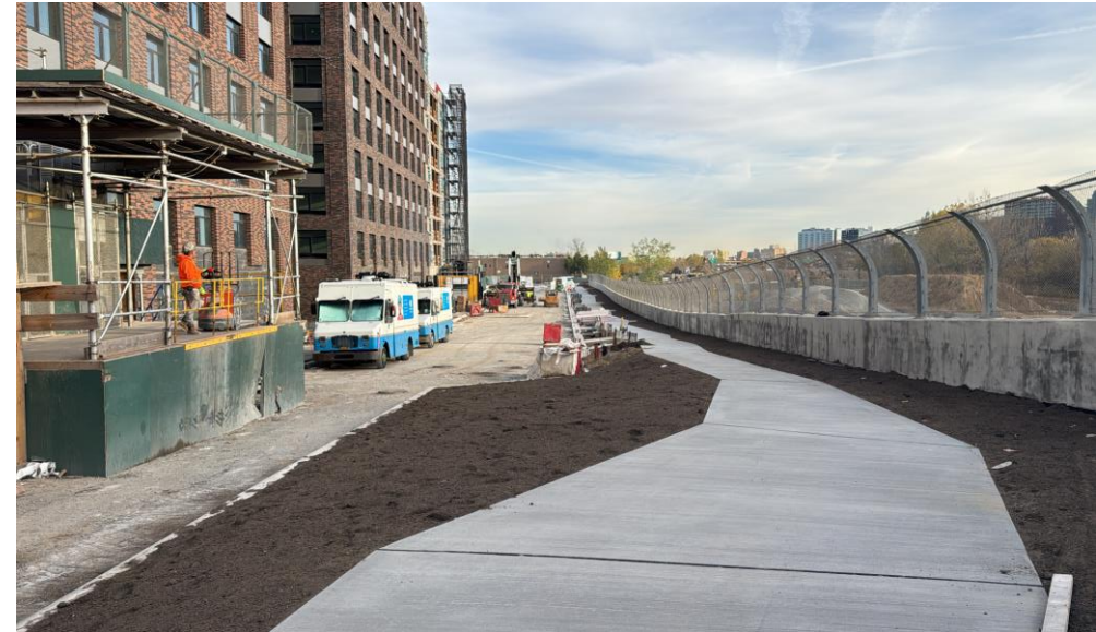
39 th Ave Sidewalk, Bioswales, & Planting Preparation November 2025
