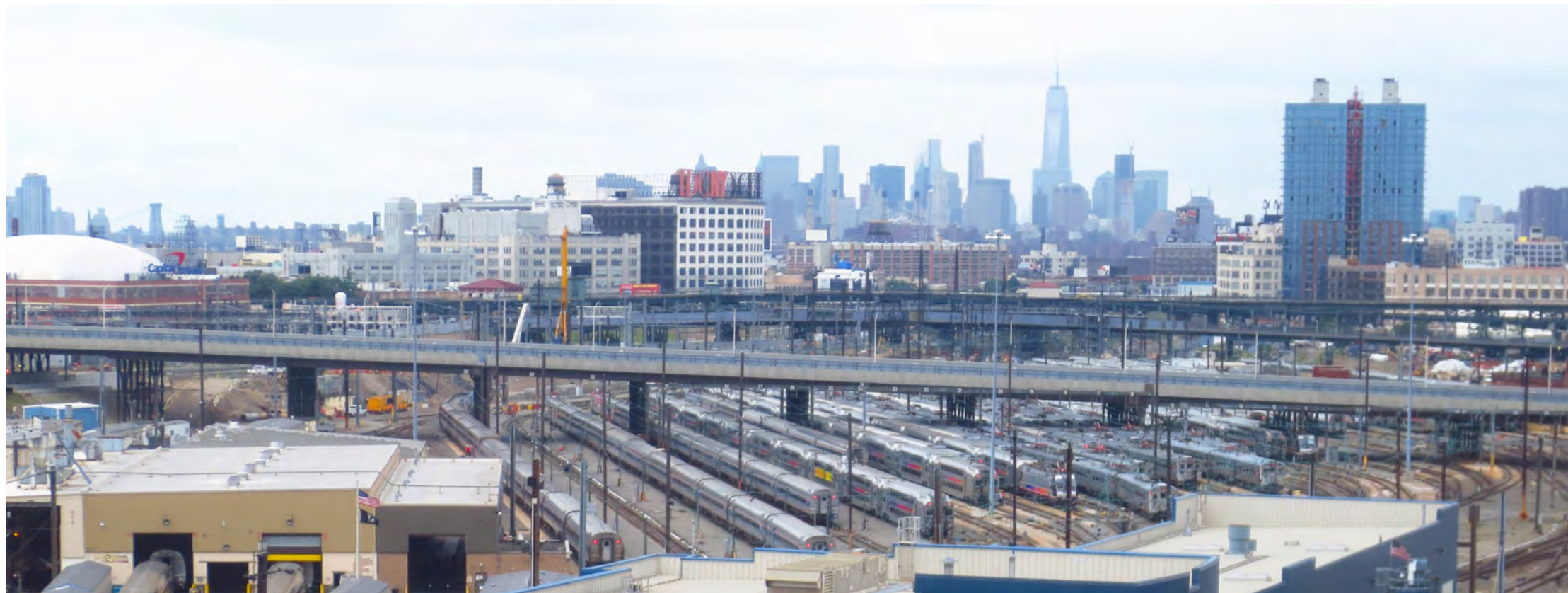
FIGURE 1.2: SUNNYSIDE YARD: EXISTING CONDITION
