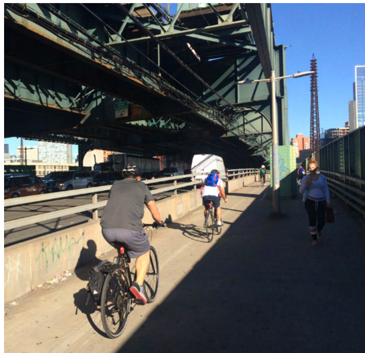
FIGURE 2.45 BIKE PATH / ED KOTCH QUEENSBOROUGH BRIDGE
