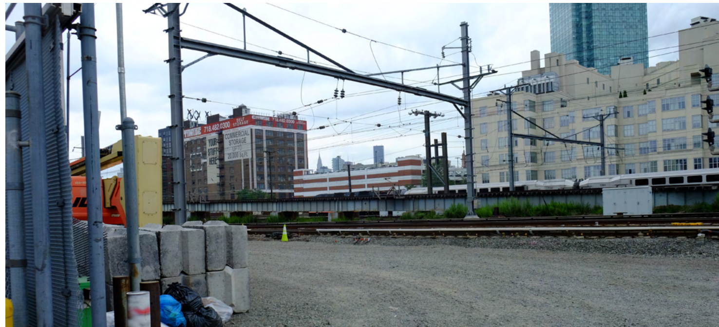
FIGURE 3.3: CATENARY PORTAL SYSTEM
