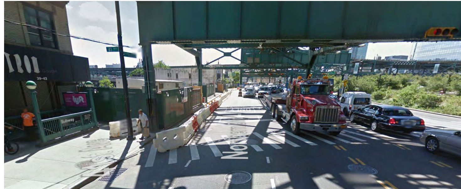
FIGURE 2.34: NORTHERN BOULEVARD AT QUEENS PLAZA STATION
