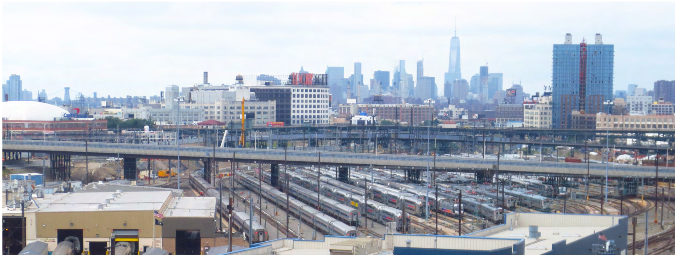
FIGURE 1.2: SUNNYSIDE YARD: EXISTING CONDITION
