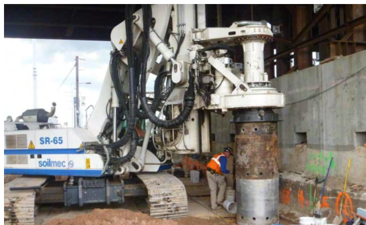
FIGURE 3.42: LOW HEADROOM PILING RIGS
