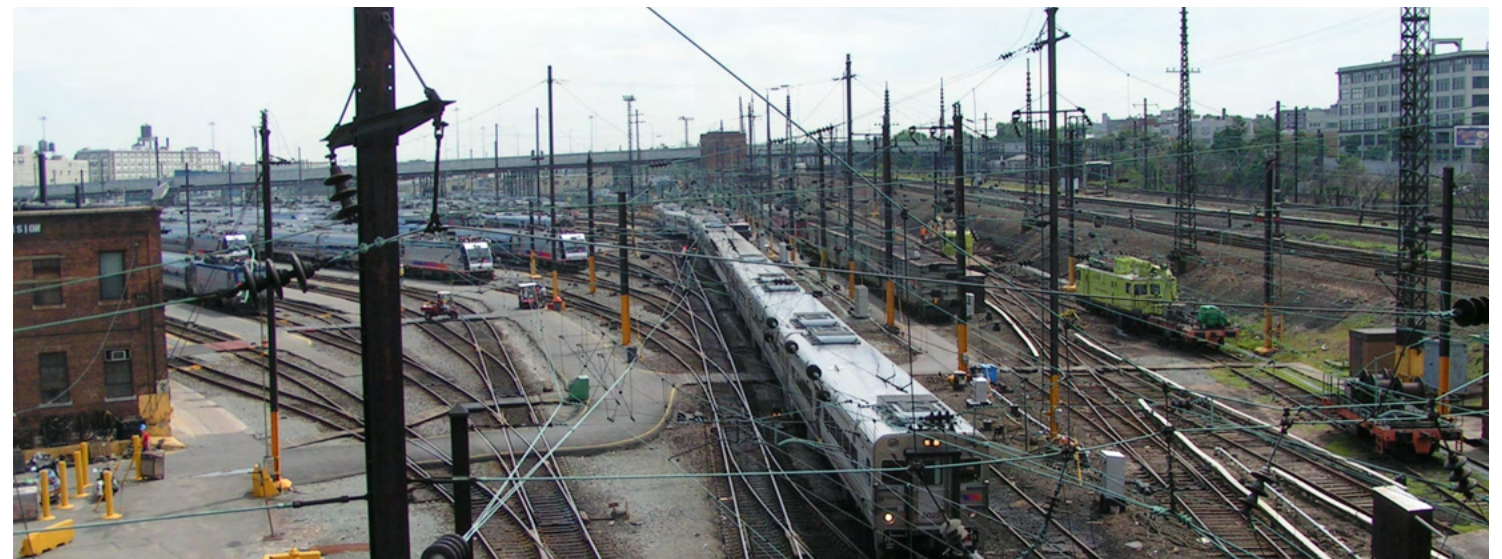
FIGURE 3.2: SUPPORT WIRES SPANNING SUNNYSIDE YARD
