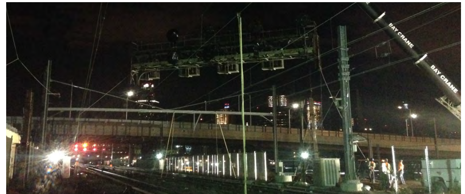
FIGURE 3.44 SIGNAL BRIDGE INSTALLATION
