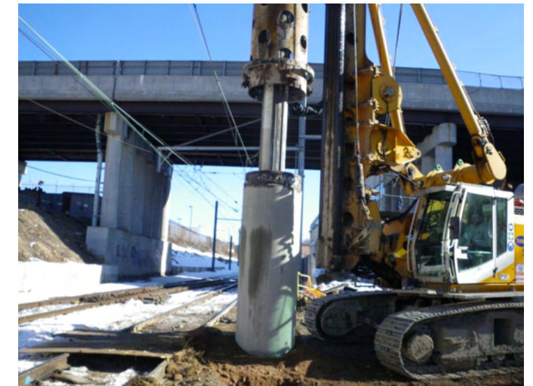
FIGURE 3.33 :SECANT PILES
