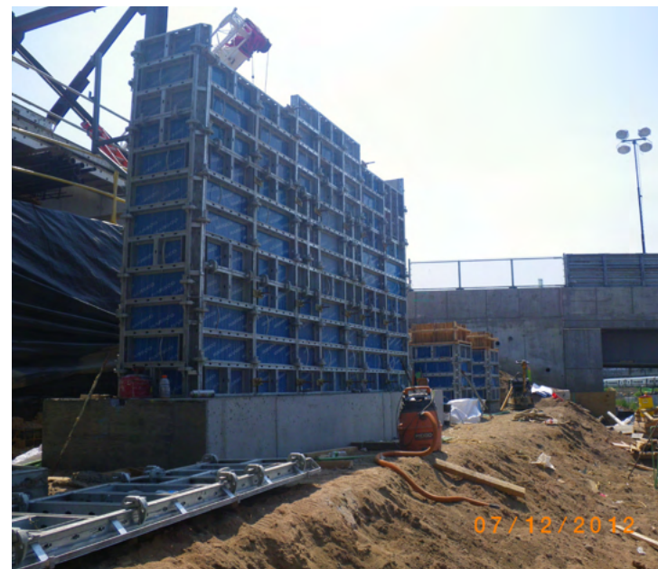
FIGURE 3.43: INTERNALLY TIED FORMWORK
