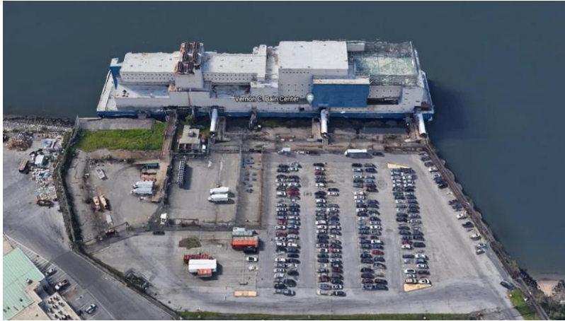
Vernon C. Bain Center (VCBC) prison barge and parking lot, circa 2021
