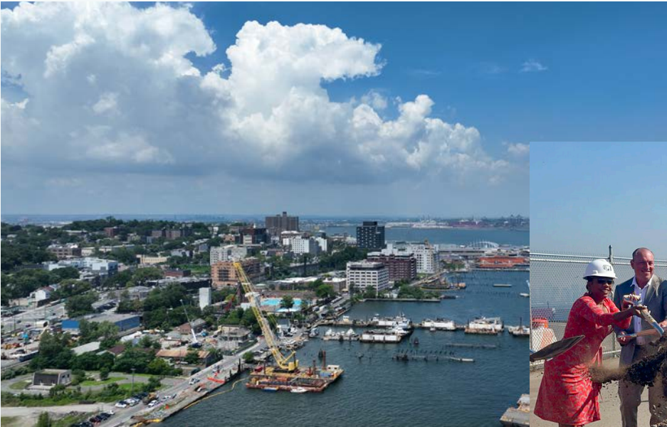
Construction at Tompkinsville Esplanade.
