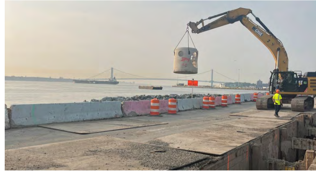
Construction underway for New Stapleton Waterfront
