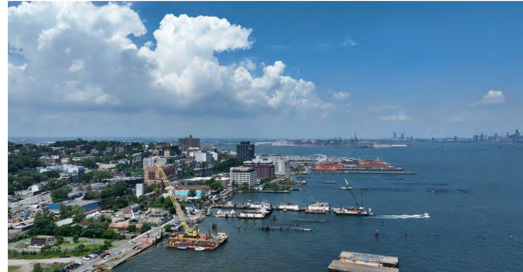
Construction of Tompkinsville Esplanade looking towards St. George
