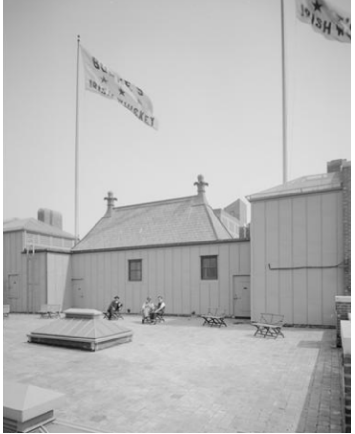
Roof of 616-620 West 46th Street (1912)
