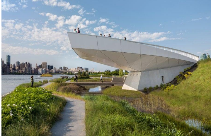
Resilient Waterfront Walkway at Hunter's Point South
