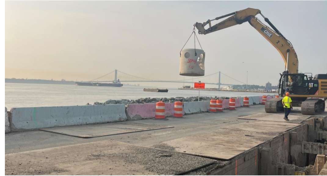
Construction underway for New Stapleton Waterfront
