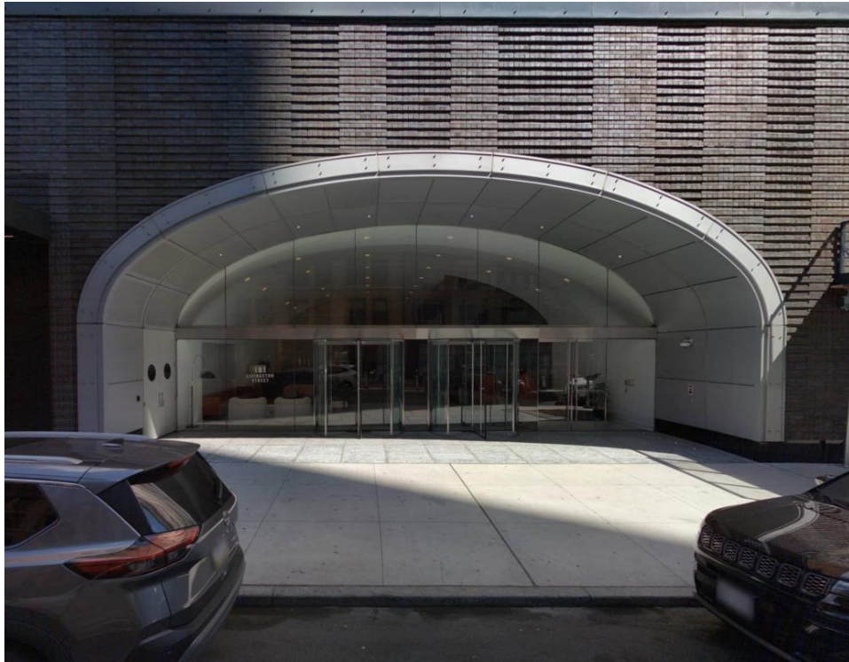
Figure 3: The Wheeler – Existing Lobby Entrance at 181 Livingston Street
