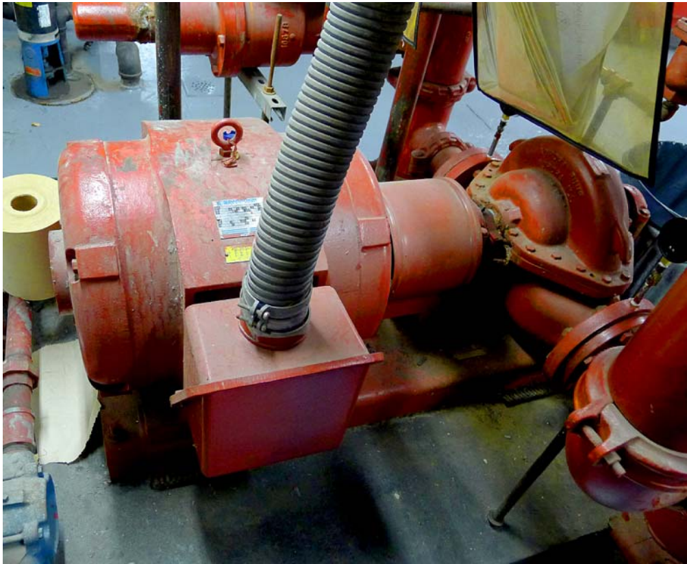
12 FP - Fire Pump ROOM LOCATION : BOILER ROOM FLOOR LOC. : BASEMENT
