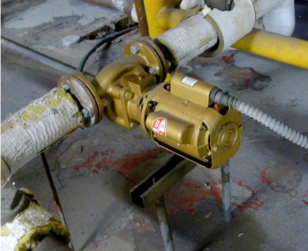
14 CP-1 - Circulating Pump no. 1 ROOM LOCATION : BOILER ROOM FLOOR LOC. : BASEMENT
