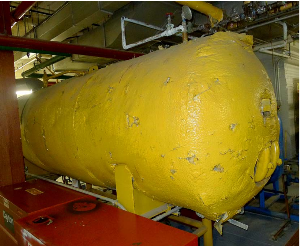
3 DHWST - Domestic Hot Water Storage Tank ROOM LOCATION : BOILER ROOM FLOOR LOC. : BASEMENT
