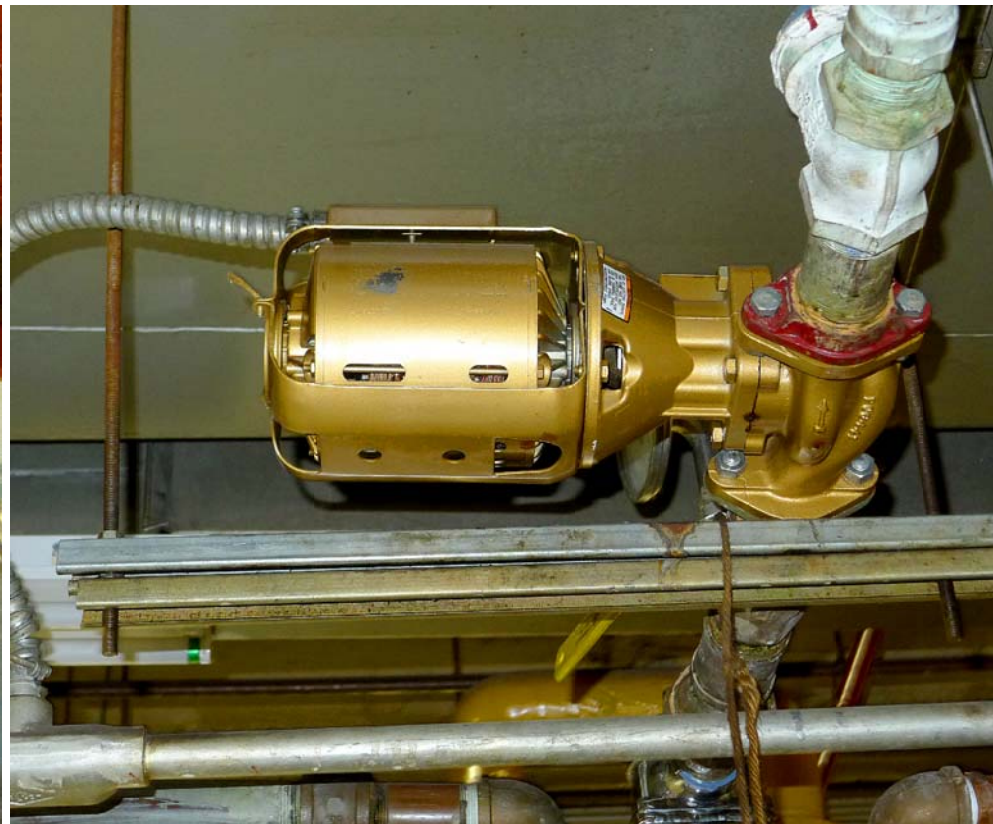
10 CP(o) - Circulating Pump (overhead) ROOM LOCATION : BOILER ROOM FLOOR LOC. : BASEMENT
