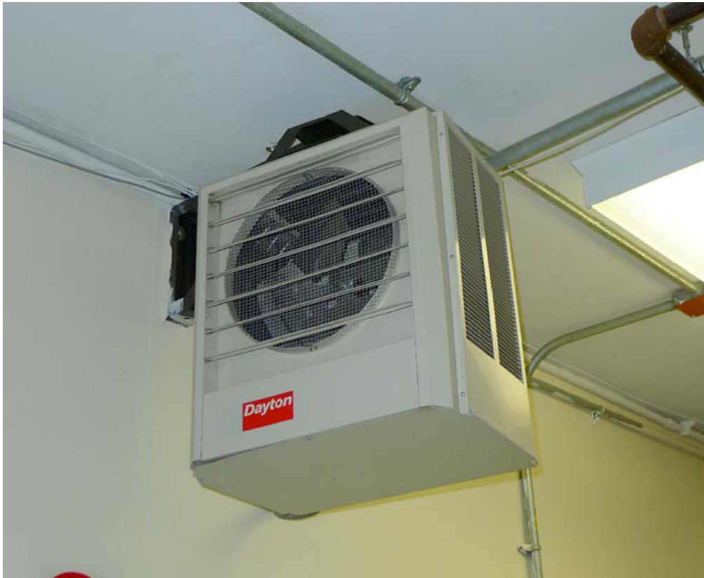
17 UH - Unit Heater ROOM LOCATION : DINING FLOOR LOC. : 1F
