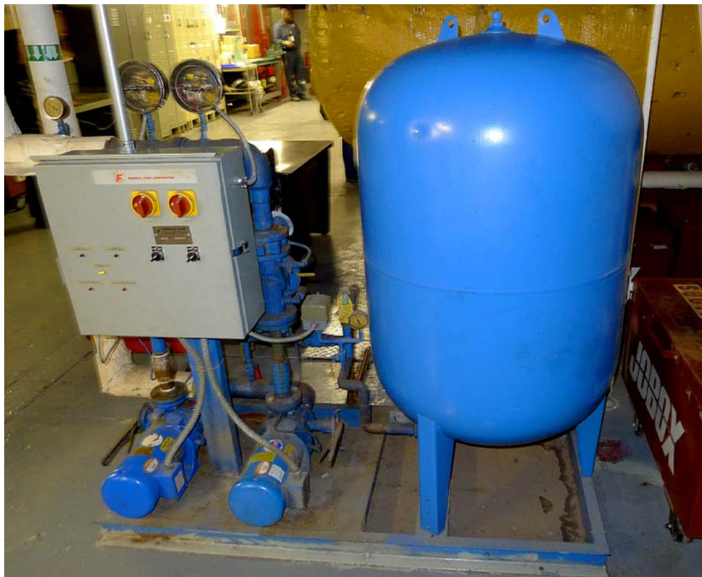
6 DBP - Duplex Domestic Booster Pump Set ROOM LOCATION : BOILER ROOM FLOOR LOC. : BASEMENT
