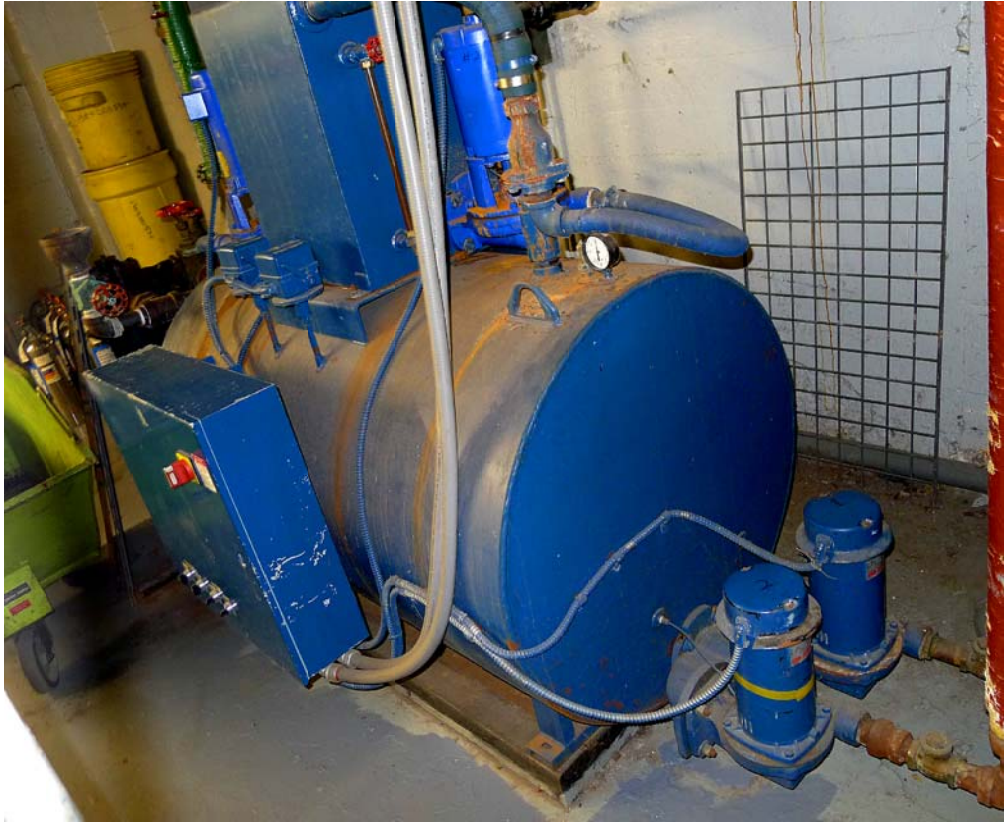
5 BF - Boiler Vacuum Feed Pumps & Tank ROOM LOCATION : BOILER ROOM FLOOR LOC. : BASEMENT
