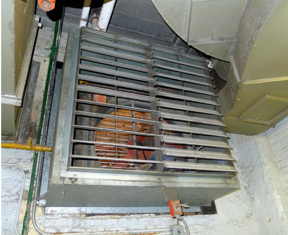
15 D - Combustion Air Damper and Fan ROOM LOCATION : BOILER ROOM FLOOR LOC. : BASEMENT
