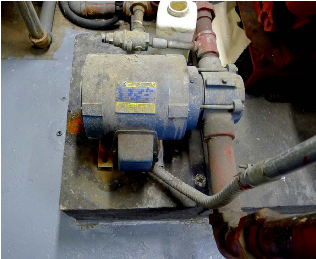
13 JP - Jockey Pump ROOM LOCATION : BOILER ROOM FLOOR LOC. : BASEMENT
