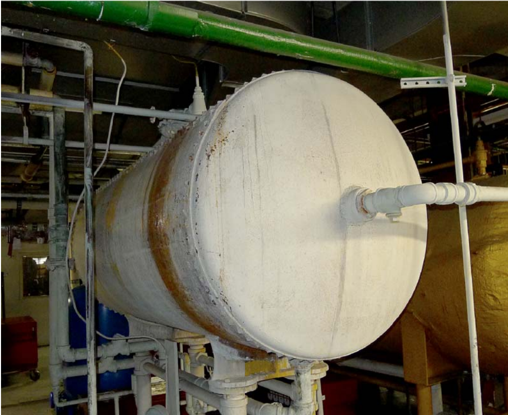
4 DWST - Domestic Water Storage Tank ROOM LOCATION : BOILER ROOM FLOOR LOC. : BASEMENT
