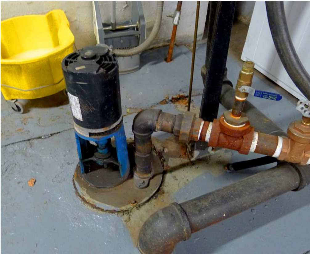
11 SEP - Sewage Ejector Pump ROOM LOCATION : BOILER ROOM FLOOR LOC. : BASEMENT
