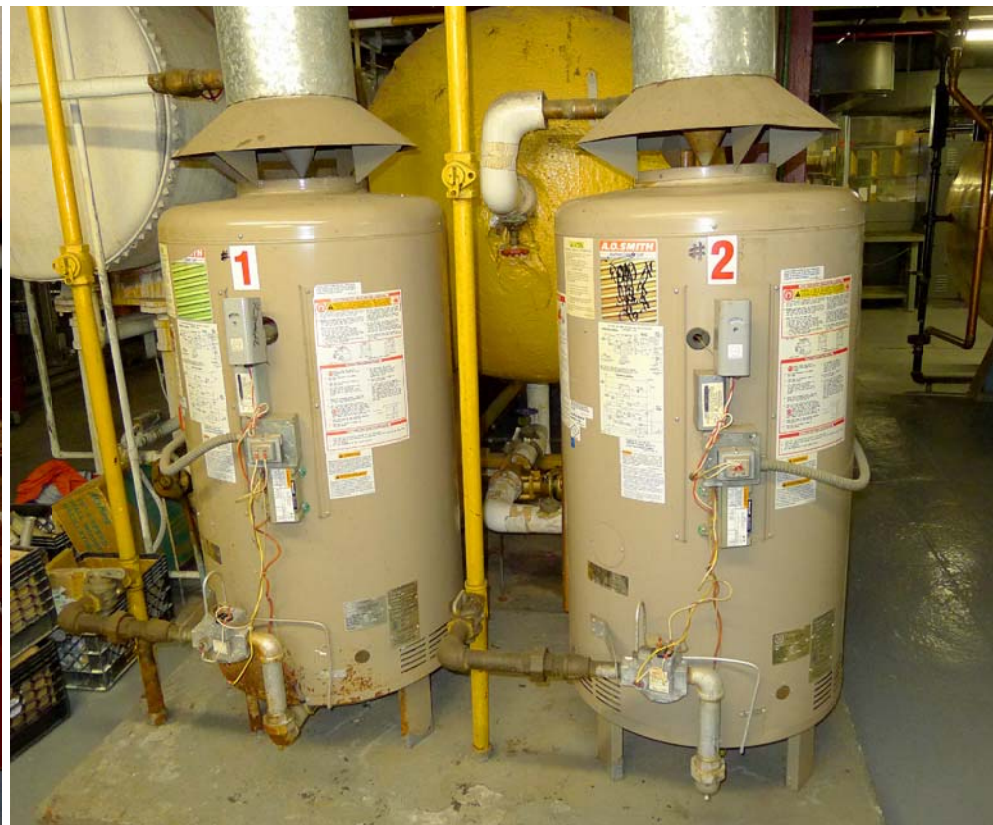
7 DWH-1~2 - Domestic Hot Water Heater nos. 1~2 ROOM LOCATION : BOILER ROOM FLOOR LOC. : BASEMENT
