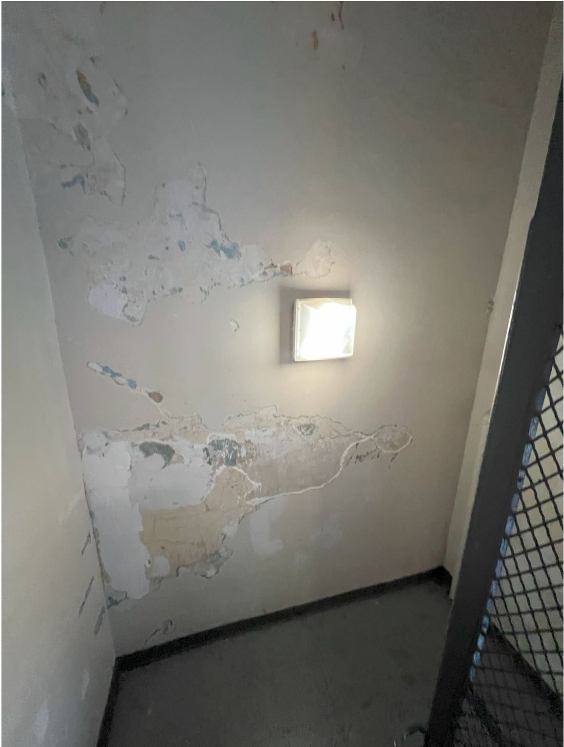
Signs of Previous Moisture Infiltration in Stairwell
