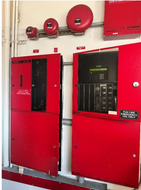
Fire Alarm Control Panel
