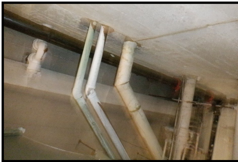
Photo #4: Suspect ACM Piping
