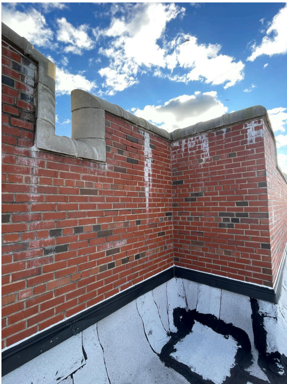
Photo 16: Efflorescence at the parapet wall; patching at roof
