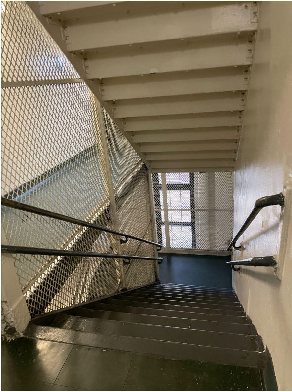
Photo 23: Cantilevered intermediate landing
