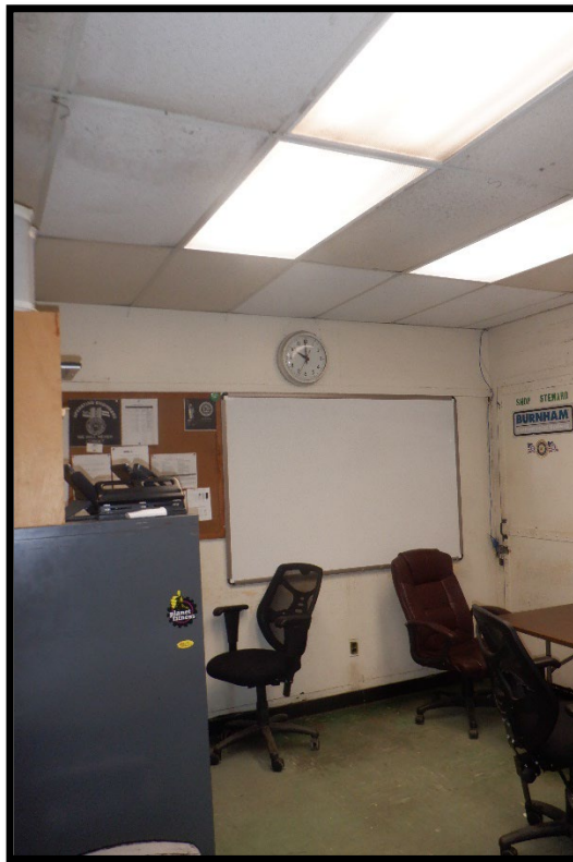
Photo #8: Suspect ACM Ceiling Tile, Sheetrock/Joint Compound
