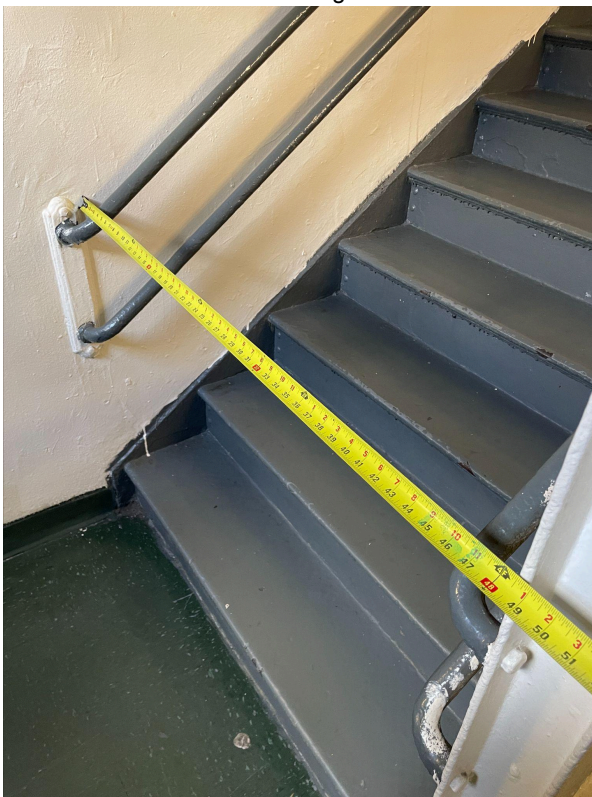
Photo 20: Stair width typically 4'-0"
