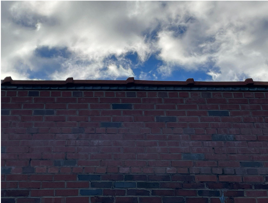
Photo 17: Renovated flashing under terracotta coping and mortar repair
