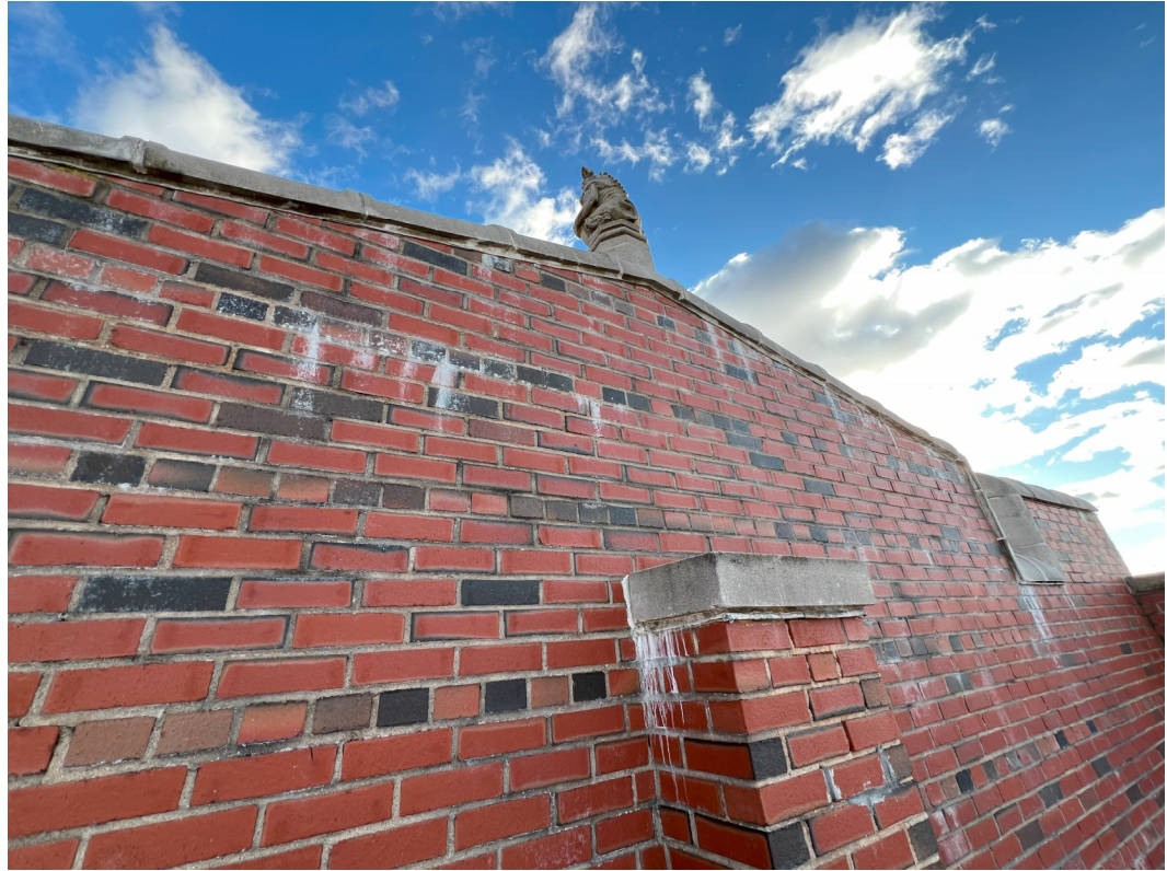
Brick Efflorescence and Mortar Deterioration
