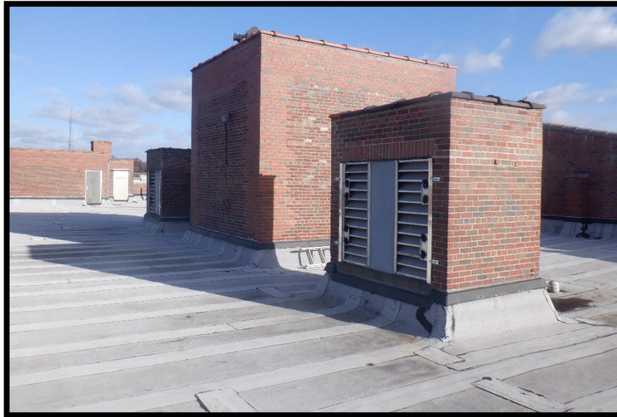
Photo #1: Suspect ACM roofing, flashing, coping stone mastic
