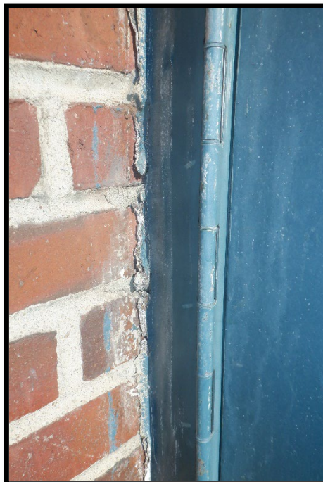
Photo #2: Suspect ACM/PCB Door Caulking
