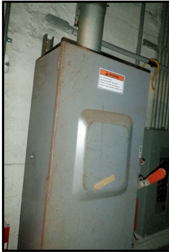
Photo #5: Suspect Electrical Box Backing
