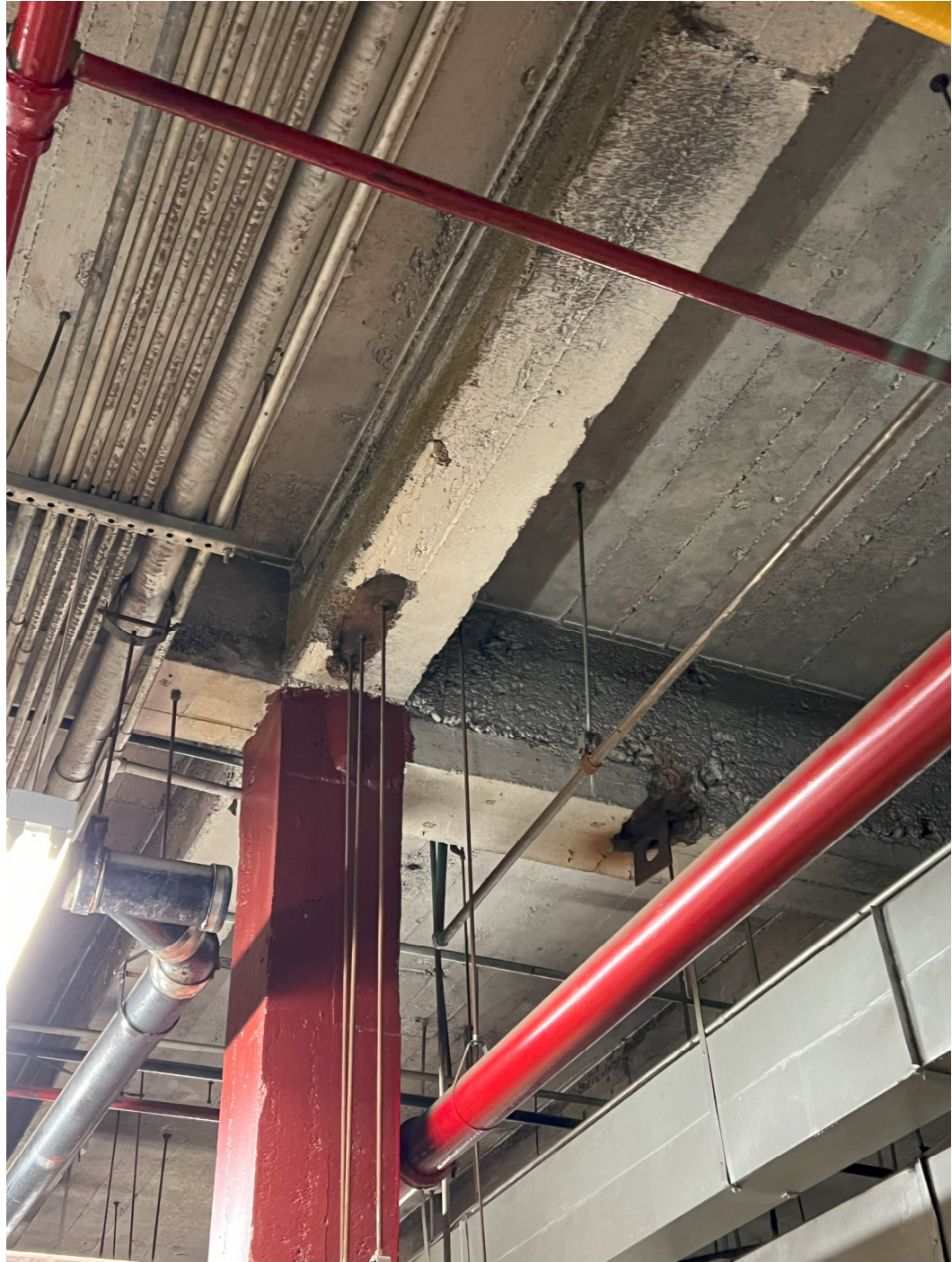
Exposed Steel Beam Soffits at MEP Hangers in Cellar
