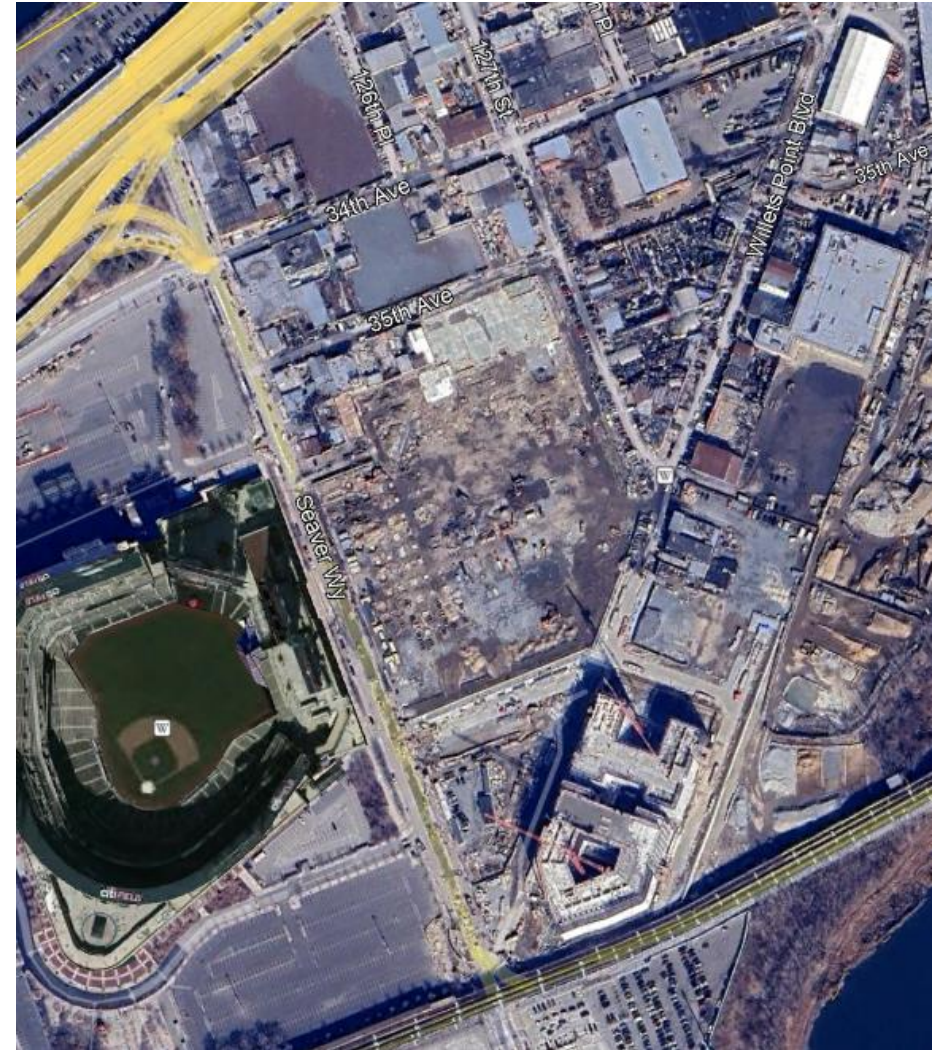
February 2025 – Remediation Complete, Building and Infrastructure Progress
