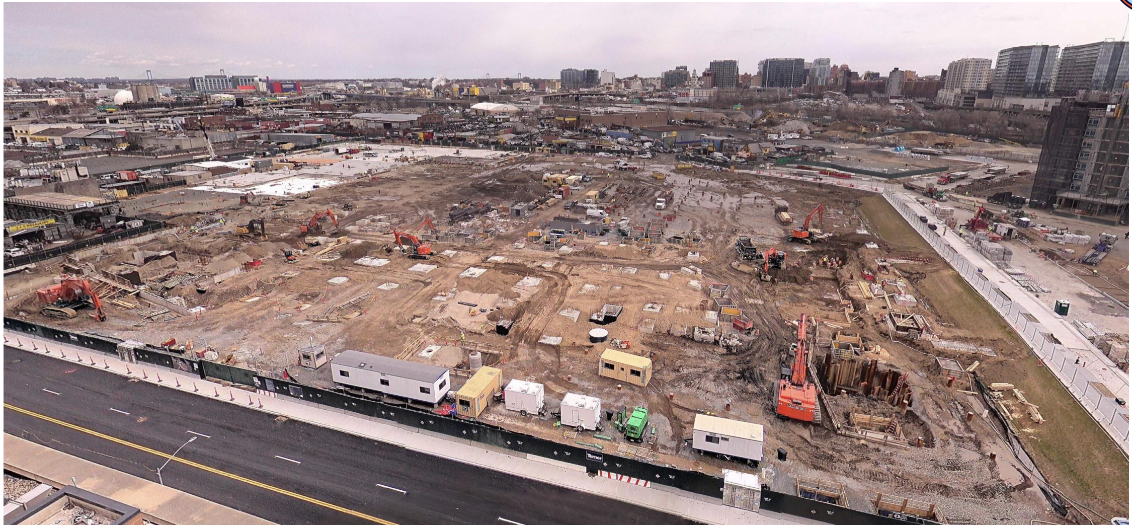
Above: Aerial photo of stadium work site (April 2025)
