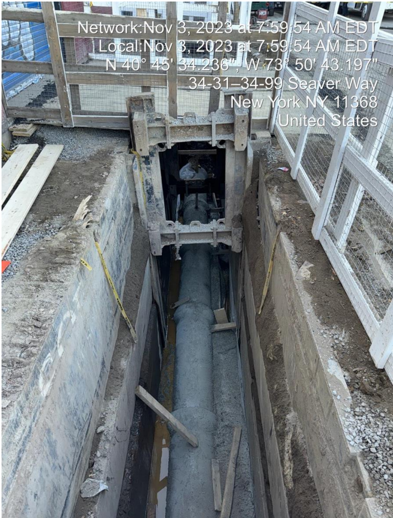
Sanitary Sewer Pipe Installation November 2023
