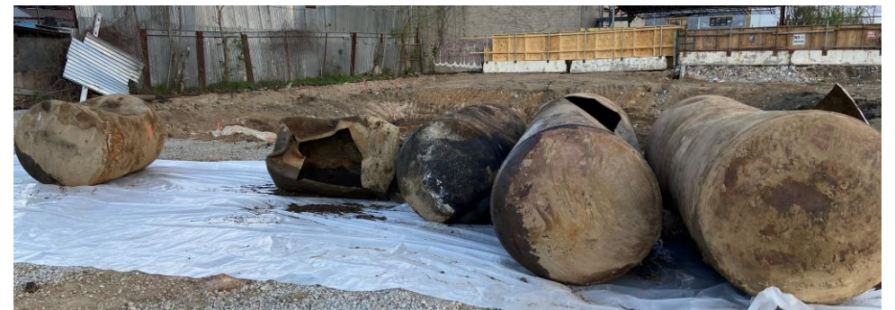
Removed Underground Fuel Storage Tanks
