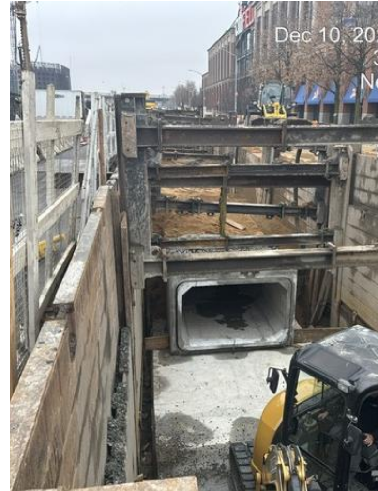
Storm Sewer Installation November 2024 to March 2025
