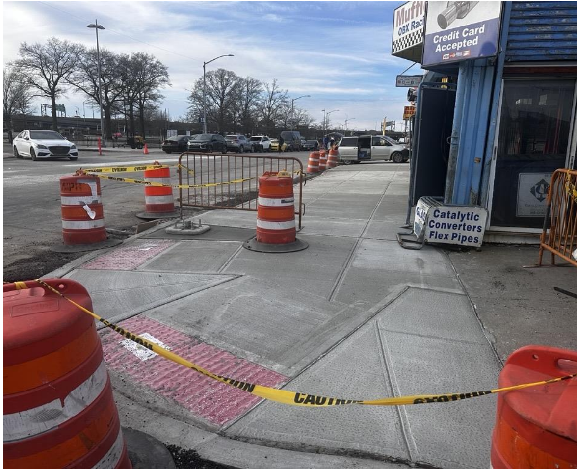
Sidewalk & Curb Restoration Near Existing Shops
