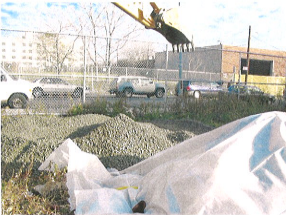
Photo 15: Backfilling the excavation with clean fill.
