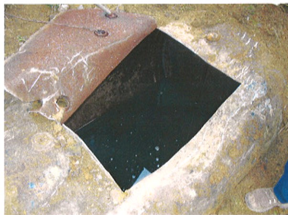
Photo 2: Top of UST cut open to inspect the contents.
