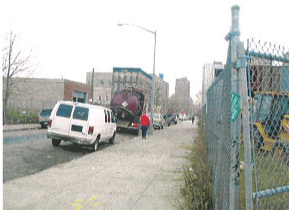
Photo 5: Vacuum truck parked on Sackman Street.
