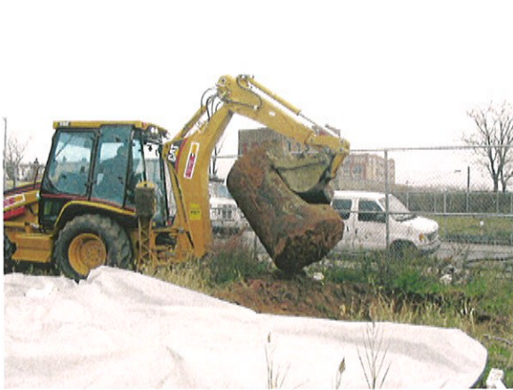
Photo 9: UST removed from ground.
