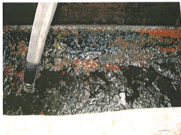
Photo 6: Pumping UST contents into vacuum truck.
