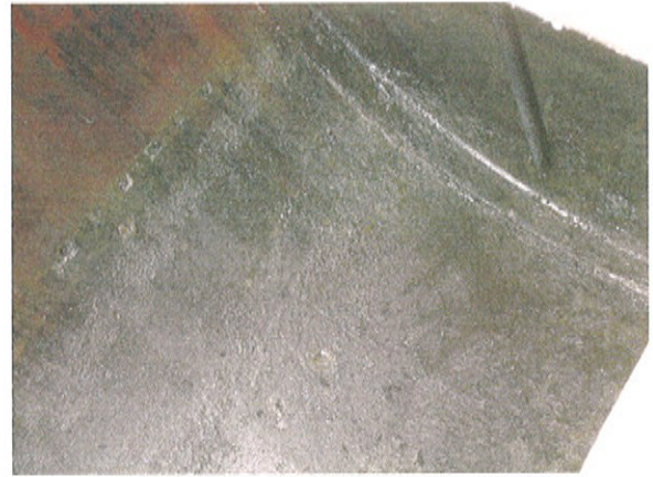
Photo 8: View of inside UST after cleaning.
