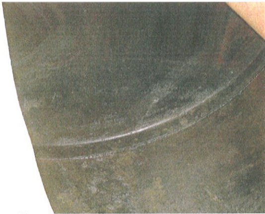
Photo 7: View of inside UST after cleaning.
