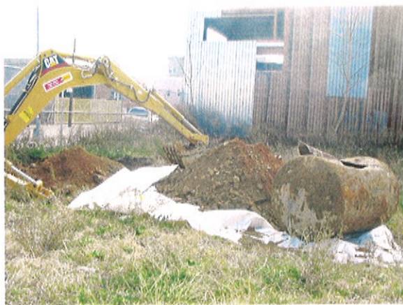
Photo 11: Soil excavation after UST removal.
