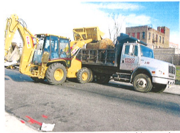
Photo 12: Loading the UST in the back of dump truck.
