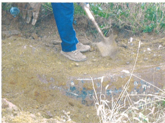
Photo 1: Overburden soil removed to expose UST.
