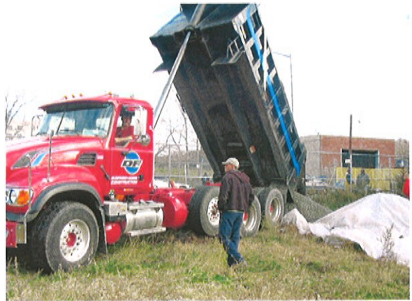
Photo 14: Truck unloading clean certified backfill.
