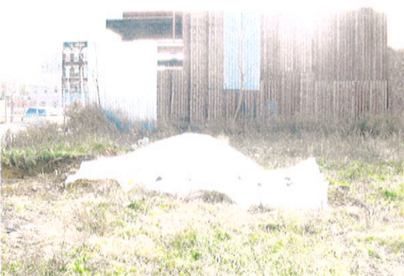
Photo 13: Excavated soil covered with plastic sheeting.
