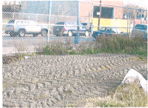
Photo 16: Backfill operation complete.
