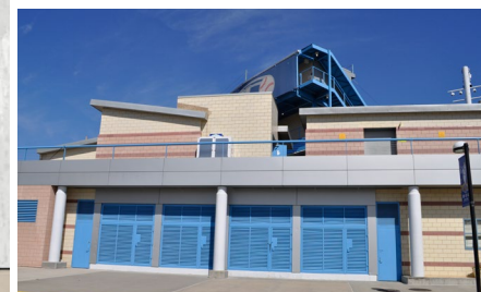
7 Vents to Transformer Room
