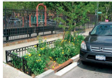
NYC Green Infrastructure Swales
