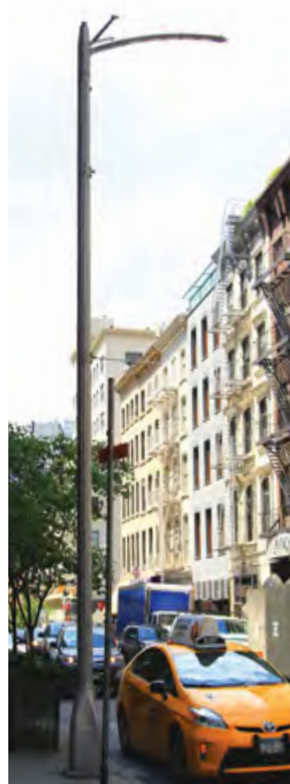
DOT Standard, City Light Fixture and Pole
