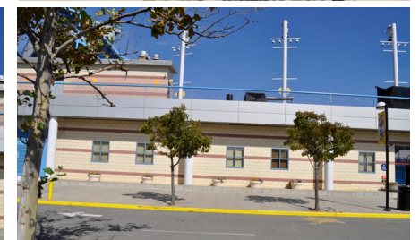
8 Windows to Offices
