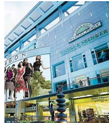
Blank walls of upper floors with signage and architectural treatment appropriate for a Perimeter Facade Siam Paragon Shopping Centre, Singapore
