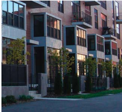
Articulated buildings that employ variety in materials and volumetric manipulations create a human scale at the lower base
