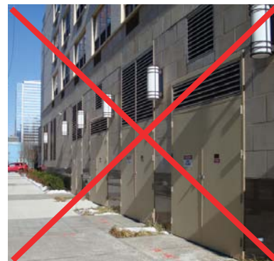
Example of a long sequence of poorly integrated service doors and grilles that create an unfriendly streetscape
