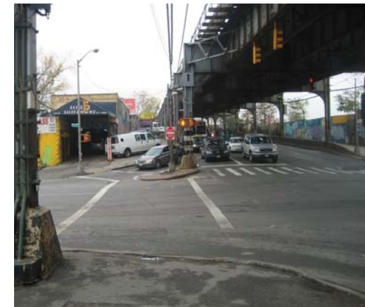
Existing condition at the intersection of Roosevelt Avenue and 126th Street, showing the elevated subway structure
