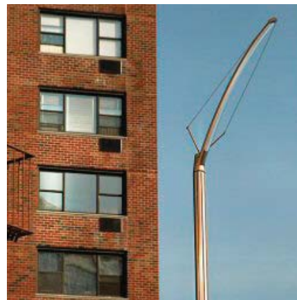
The new NYCDOT street light with LEDs, designed by Thomas Phifer and Partners
