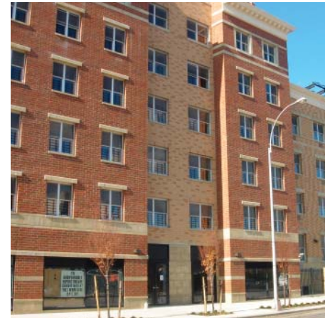
Intervale Green, Bronx Successful example of variations in material coordinated with vertical facade recesses
