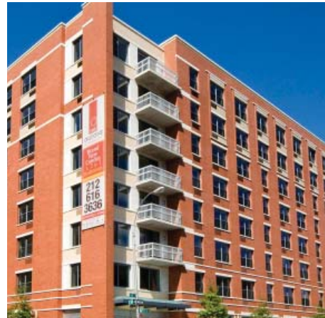
The Aurora, Bronx Successful example of the use of material changes and partially recessed balconies
