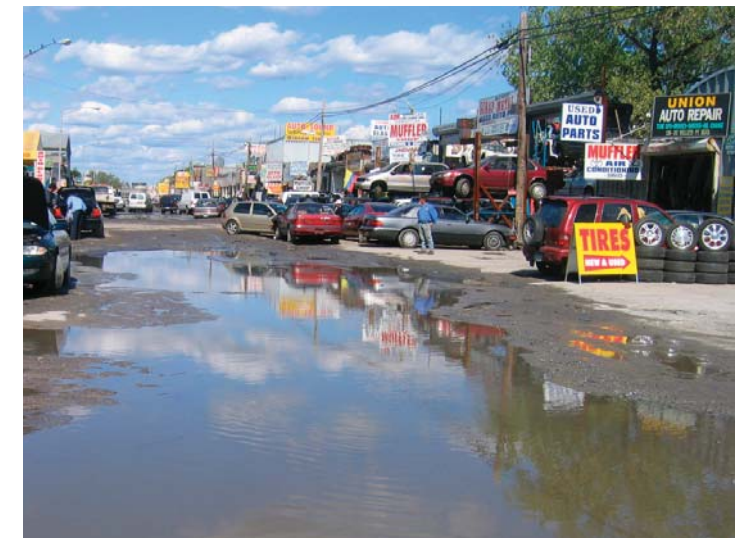
Existing conditions along Willets Point Boulevard
