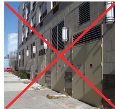
Example of a long sequence of poorly integrated service doors and grilles that create an unfriendly streetscape
