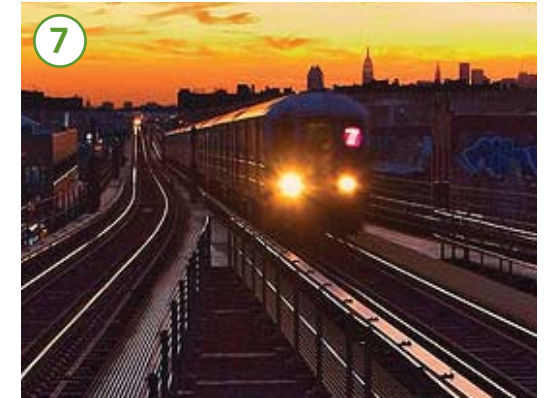
View of the elevated 7 subway line
