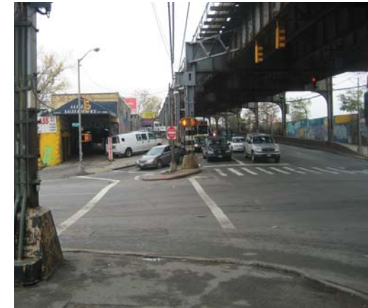
Existing condition at the intersection of Roosevelt Avenue and 126th Street, showing the elevated subway structure
