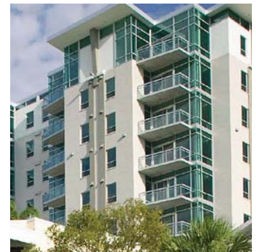
Balconies should be partially or entirely recessed into the plane of the facade or within a reentrant building corner
