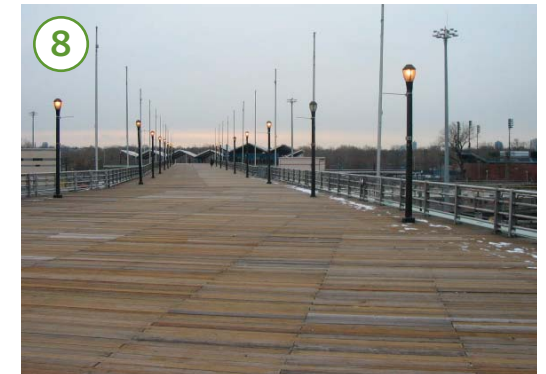
View of the Pasarella to the Long Island Railroad and Flushing Meadows Corona Park
