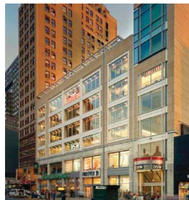
Highly transparent facade appropriate for an Internal Facade Union Square, Manhattan
