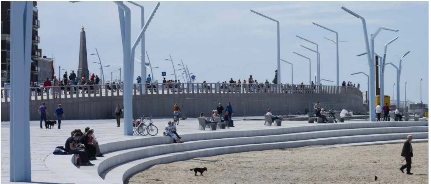
Figure 4: Multi-purpose flood protection provides safety to the coastal city of Scheveningen. Source: Mi Modern Architecture.
