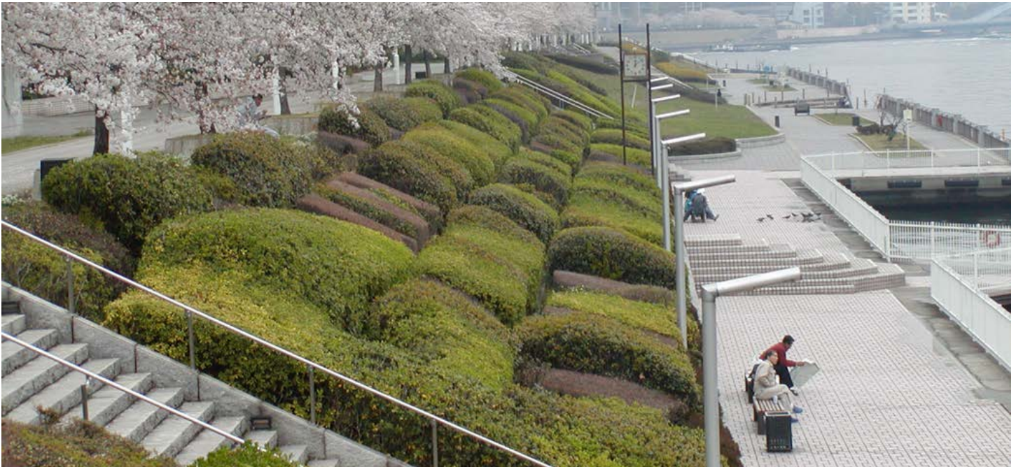
Figure 5: Example of a super levee in Japan. Source: Asian Network of Major Cities 21
