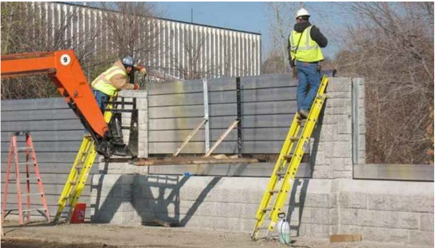
Figure 19: Example of deployable floodwalls. Source: Flood Control of America (FCA)
