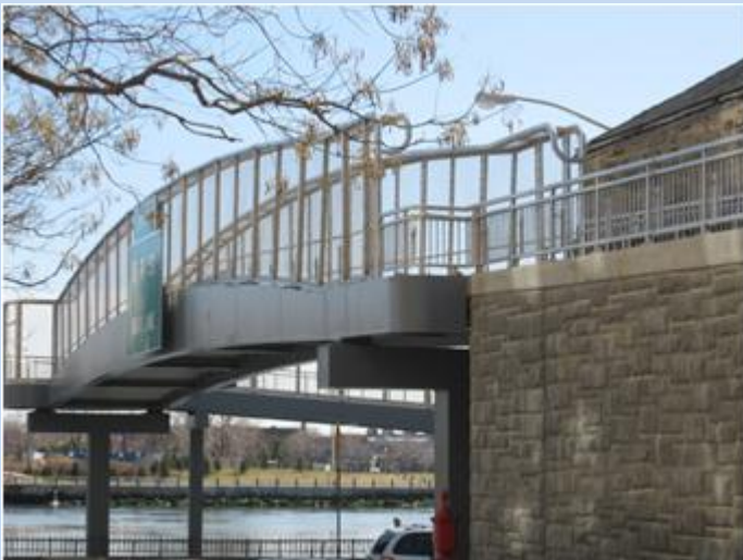
East 78 th Street Pedestrian Bridge at John Jay Park
