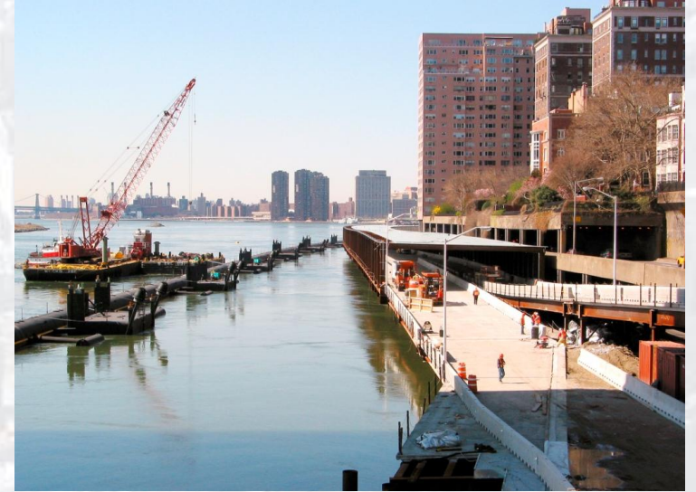
Construction of Outboard Detour Roadway (ODR)
