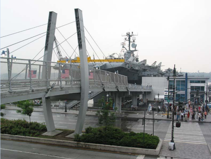
Intrepid Bridge over West Side Highway
