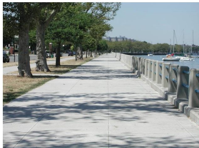
Seawall along the south side of Sheepshead Bay.
