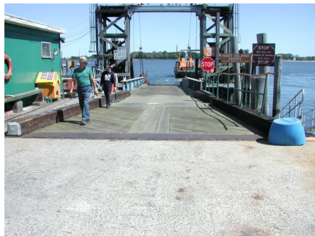
Hart Island Ferry Terminal
