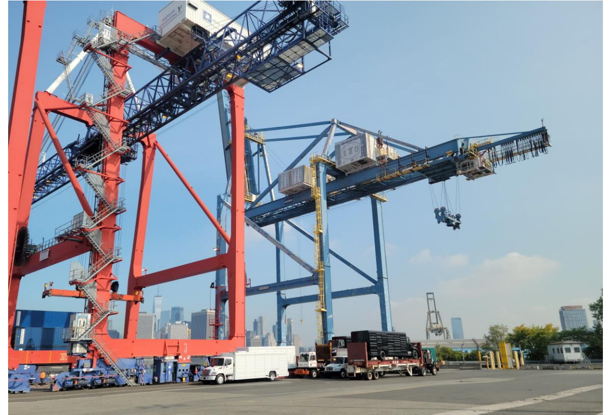
Red Hook Container Terminal Operating Cranes – Pier 10
