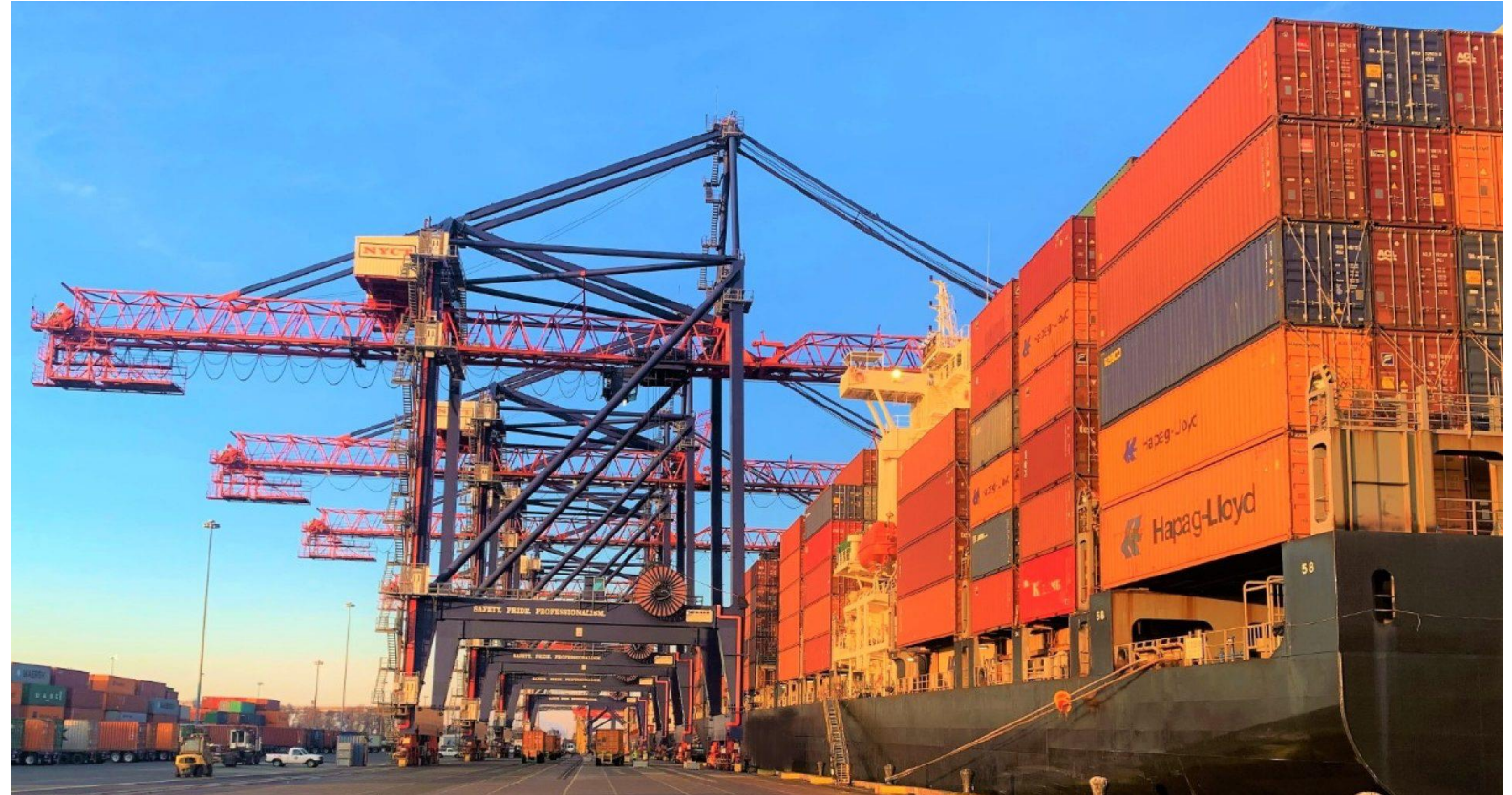
Port Liberty, Staten Island, NY – Container Cranes
