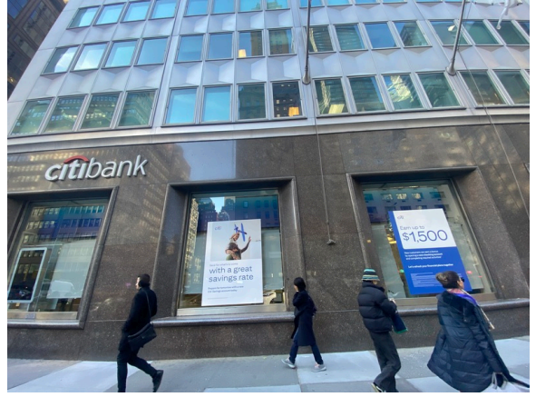
2. CitiBank Exterior (Located at Subject Property address - No interior access)
