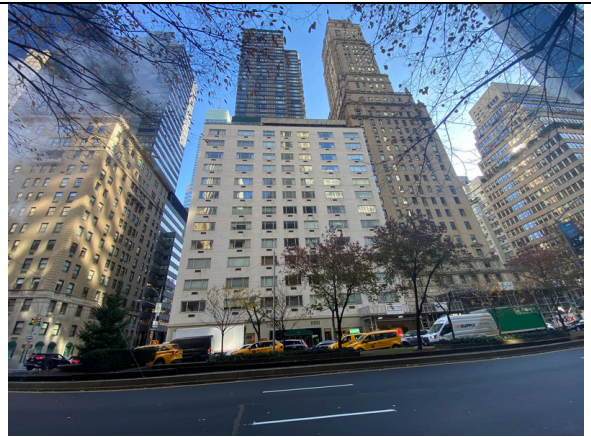
4. Mixed Use Residential and Commercial Properties adjoining to the SE across Park Avenue
