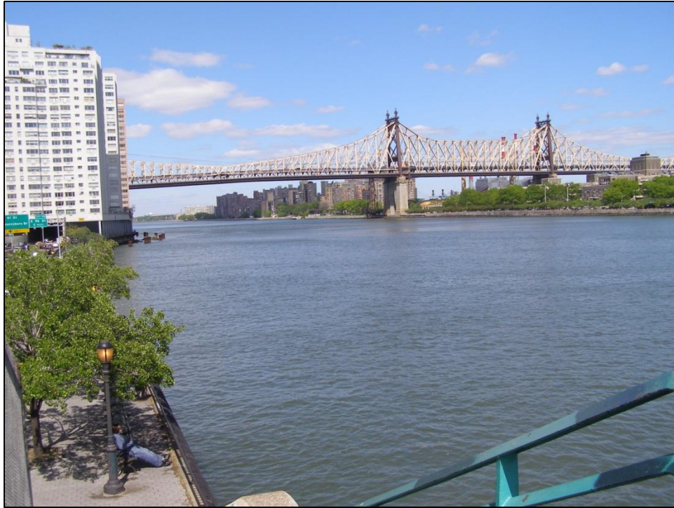
5. View looking North of the Ed Koch Queensboro Bridge from Peter Detmold Park at 51 st Street
