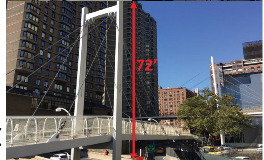
63RD STREET Span: ~125' Height: ~72'
