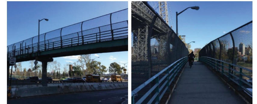
11. Pedestrian Bridge at Delancey Street
