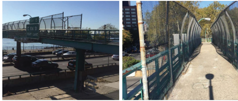
1. Pedestrian Bridge at 111th Street (Jefferson Park)
