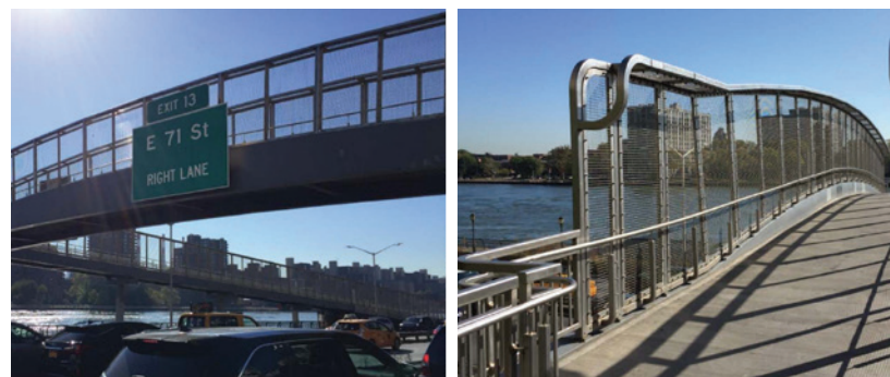
4. Pedestrian Bridge at 78th Street (John Jay Park)
