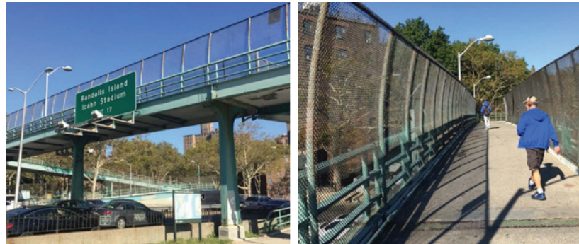
2. Pedestrian Bridge at 102nd Street (Randall's Island)
