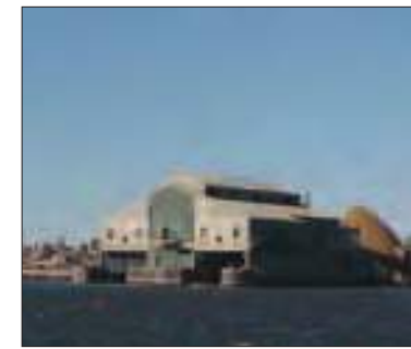
Marine Transfer Station
