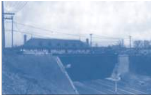
New Haven Line, Hunts Point Railroad Station
