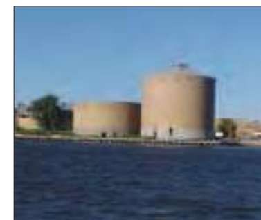
Water Pollution Control Plant
