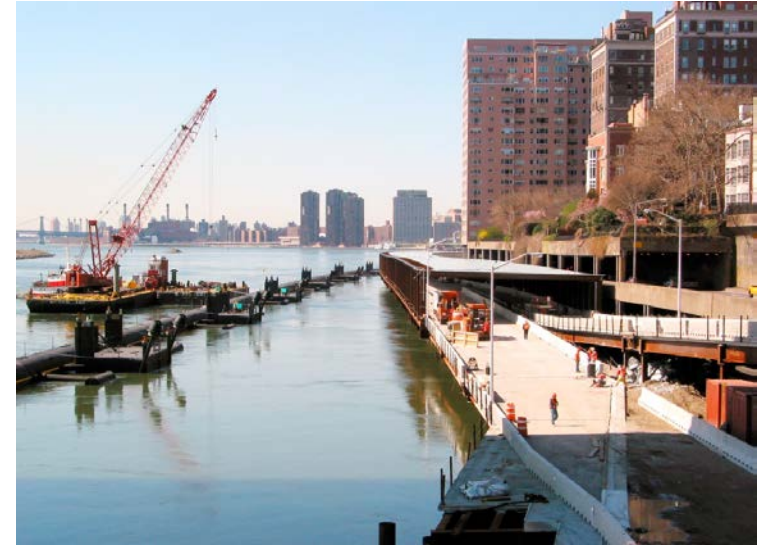
Construction of Outboard Detour Roadway (ODR)
