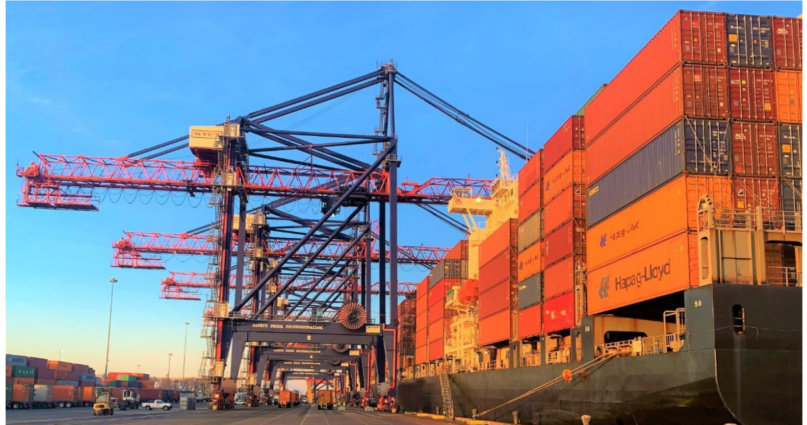
Port Liberty, Staten Island, NY – Container Cranes
