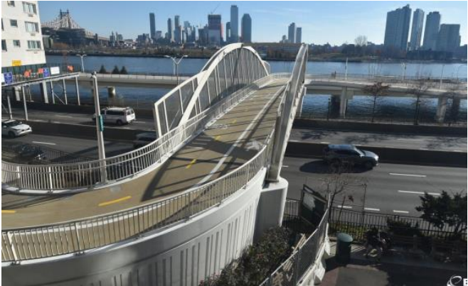
North: East Midtown Greenway & 54 th Pedestrian Bridge (Opened in 2023)
