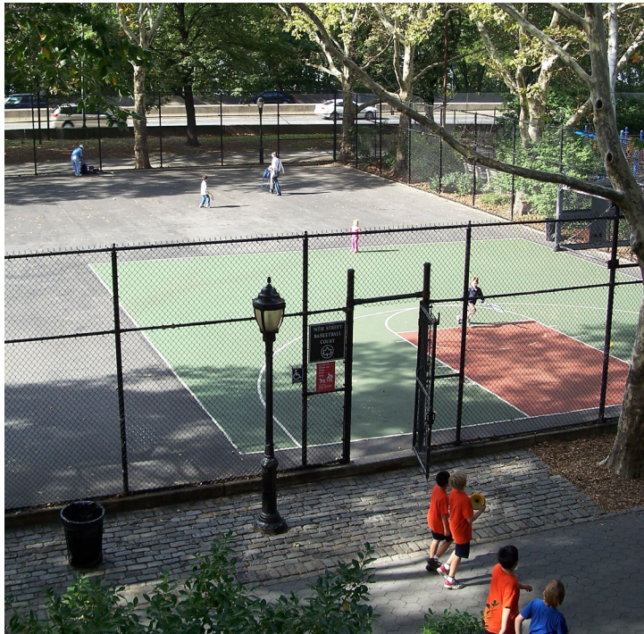
CHAIN LINK AT SPORTS COURTS - 10' HT. BLACK VINYL-COATED CLF WITH GALVANIZED POSTS PAINTED BLACK
