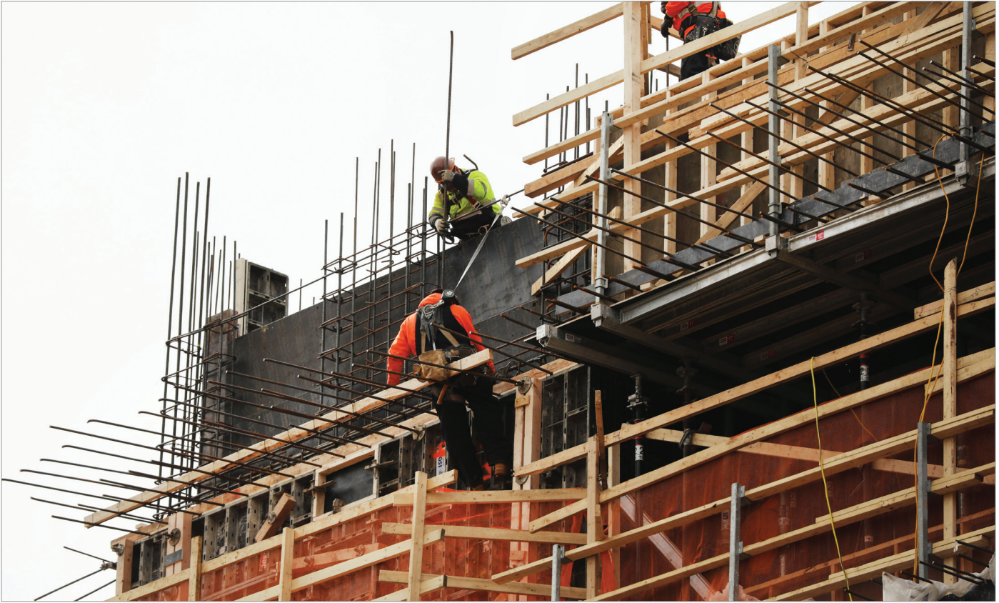
New Building Construction. Source: Getty Images
