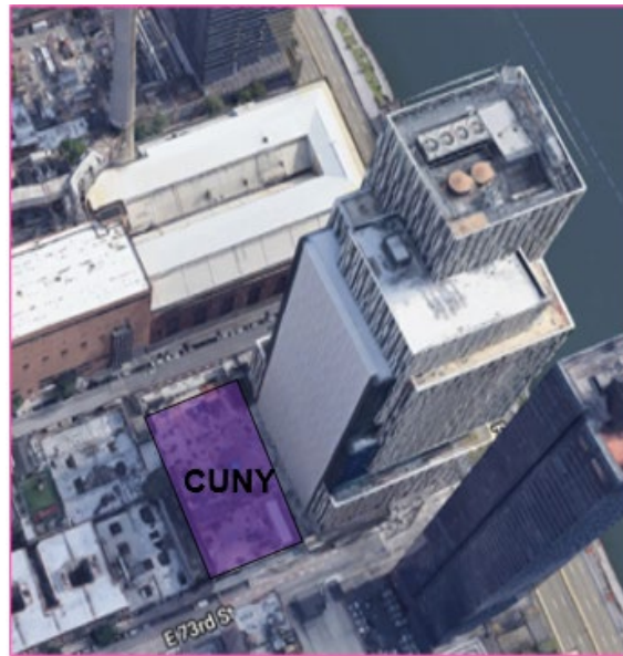
Aerial View of Site
