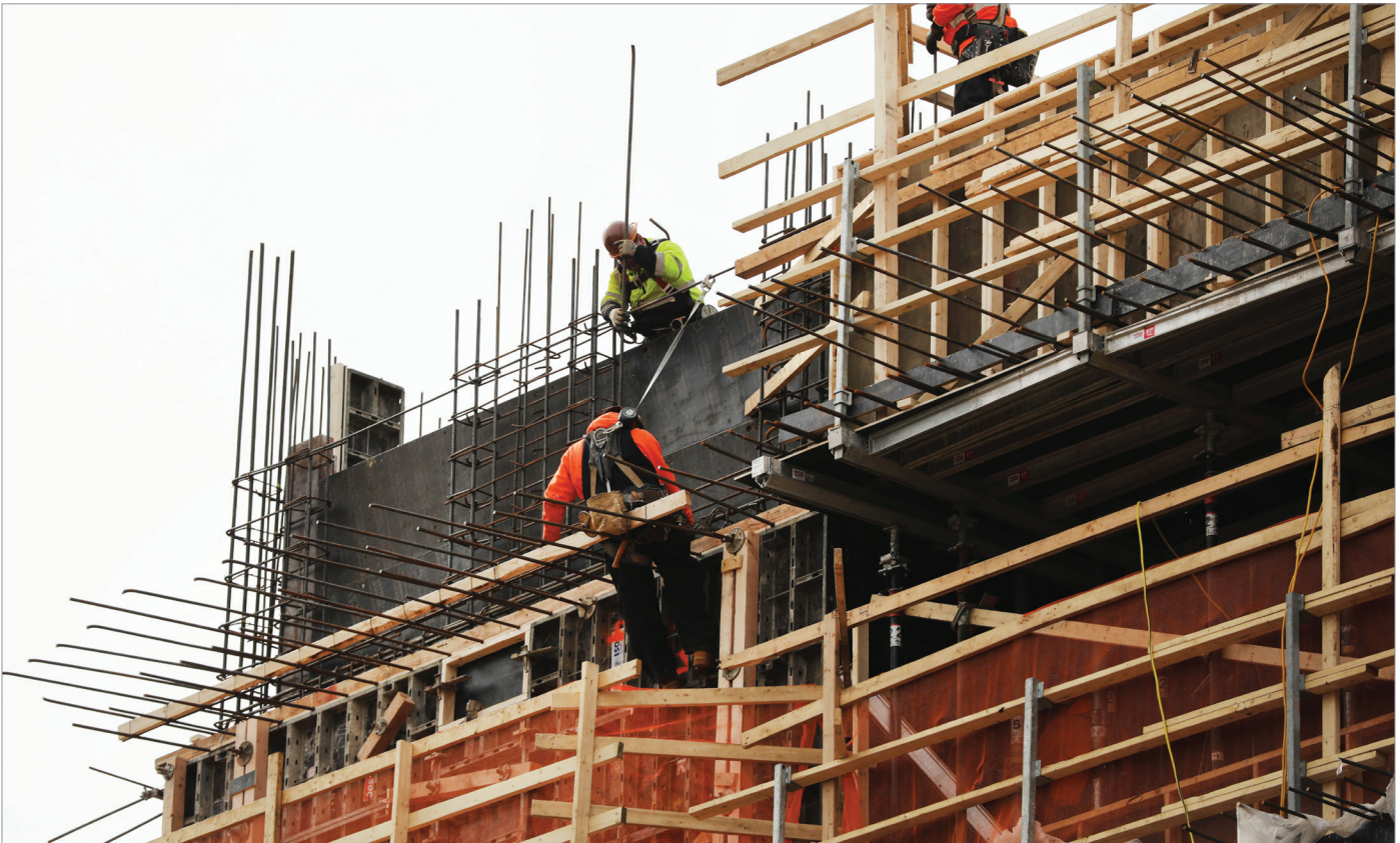
New Building Construction. Source: Getty Images
