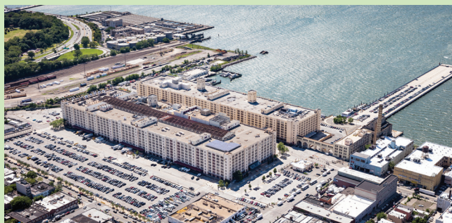
Aerial view of the Brooklyn Army Terminal. Source: Albert Vecerka
