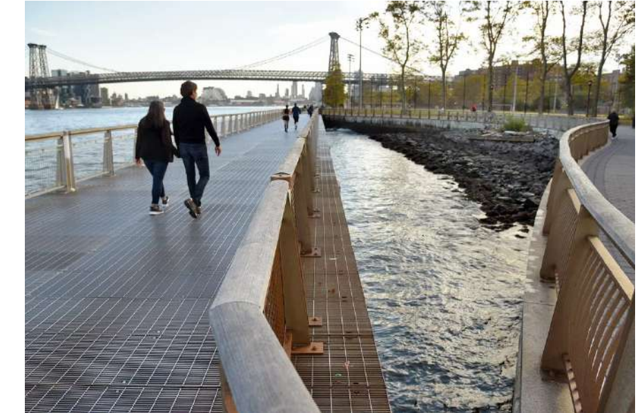
Separated Esplanade example at East River Park (Photo Credit: Nathan Kensinger)
