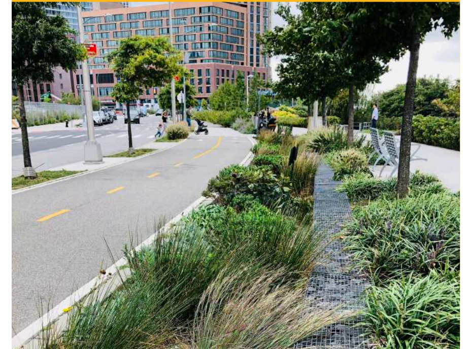
An example of green infrastructure in the form of a bioswale near a bike path at Gantry Plaza State Park (Photo Credit: Arcadis)
