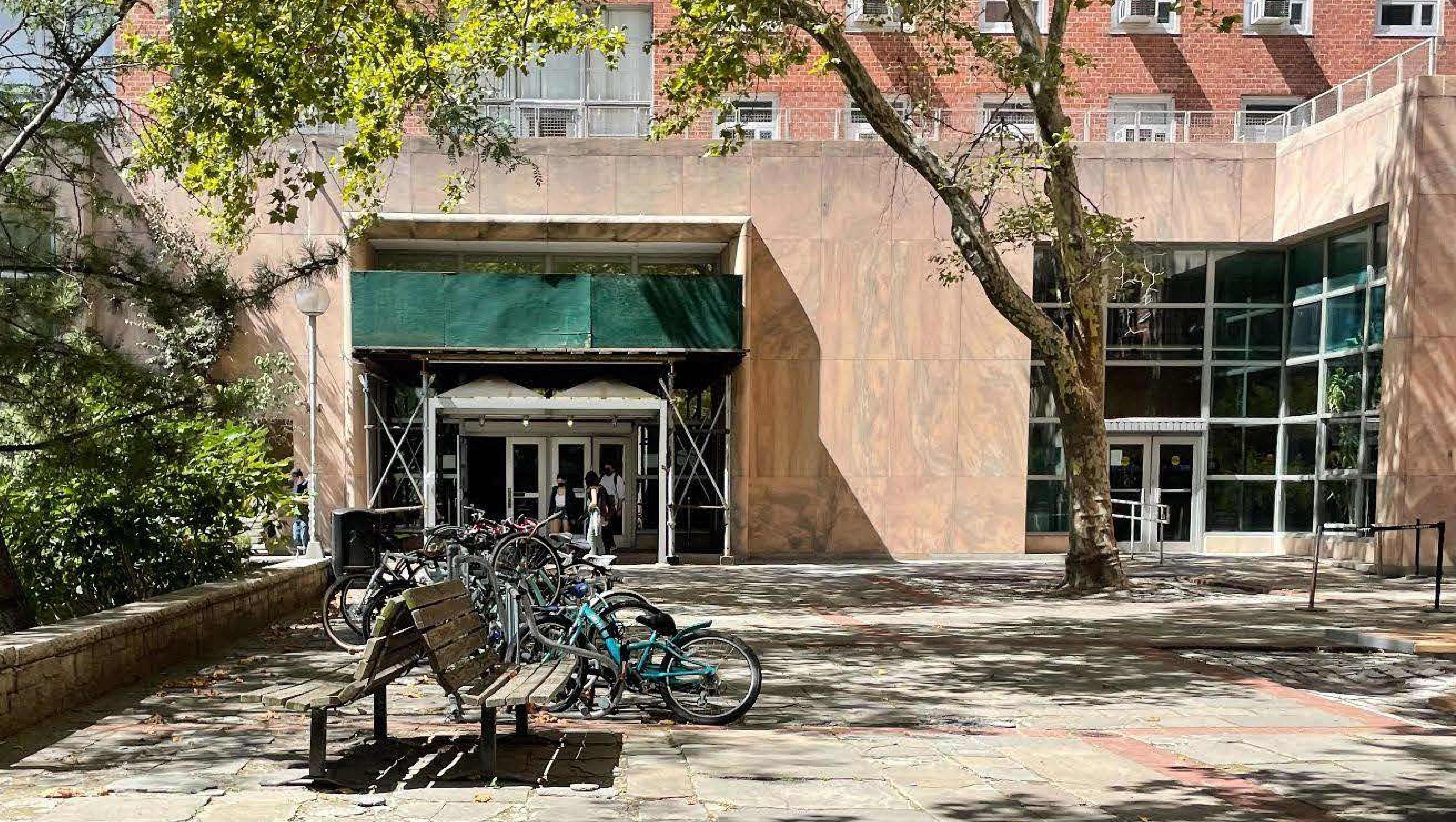
CURRENT VIEW OF CAMPUS COURTYARD & BUILDING ENTRANCE
