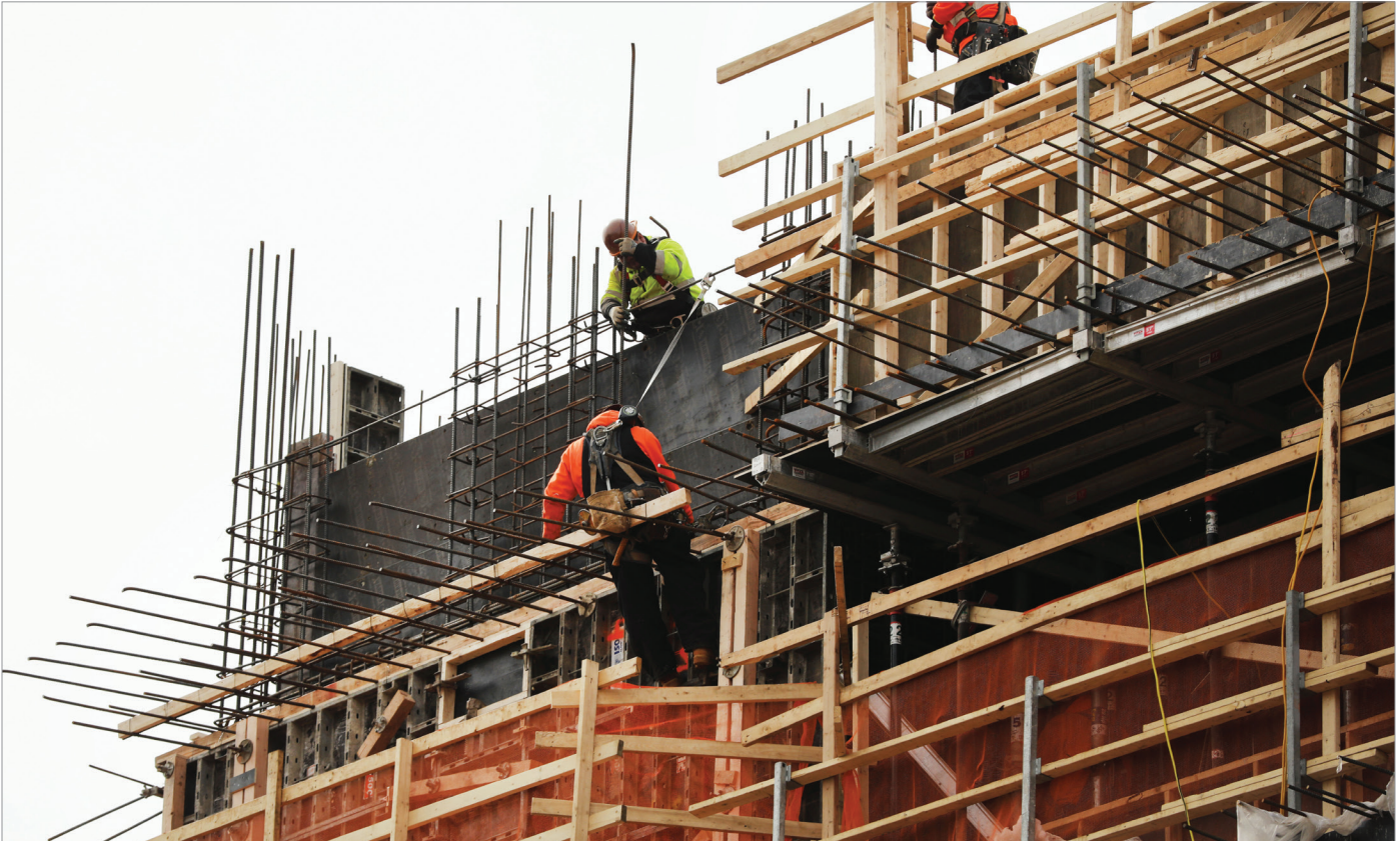
New Building Construction. Source: Getty Images
