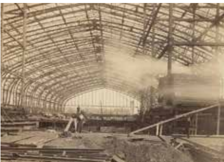
Drill hall during the construction of the Kingsbridge Armory
