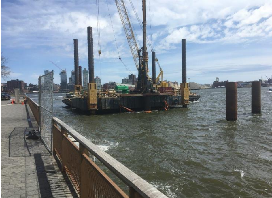
Barge mounted drill rig
