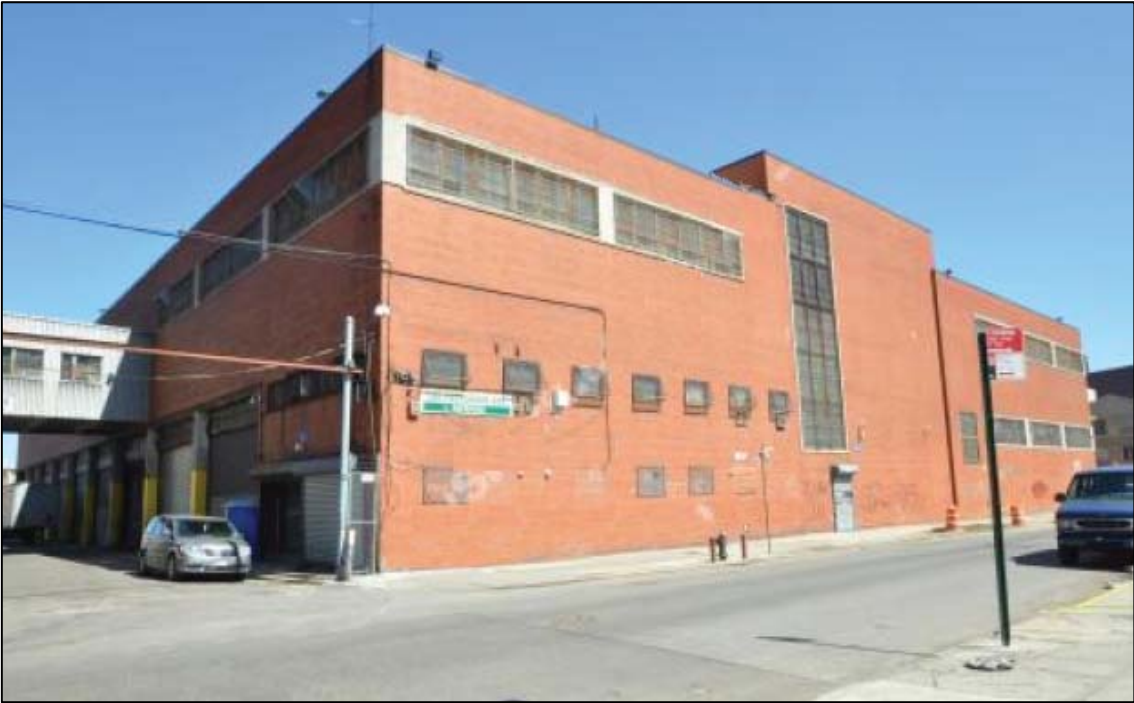
Existing Facility Photo (Former B&H Photo Warehouse)
